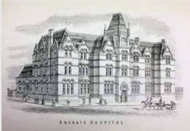
Ardwick and Ancoats Dispensary and Ancoats Hospital
