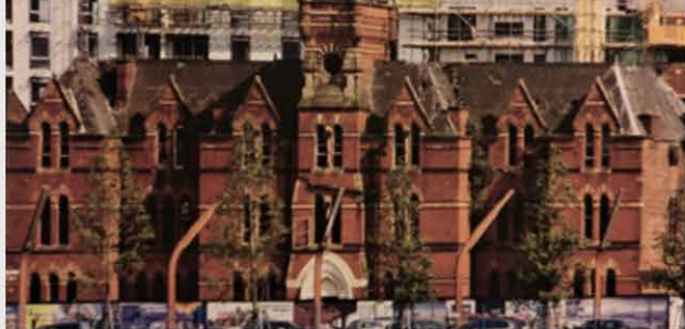
Picture showing building prior to demolition works
