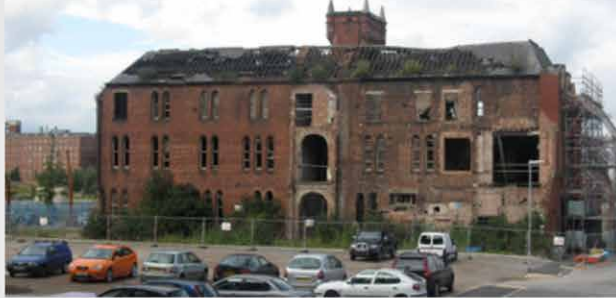
Picture showing the building with scaffolding
