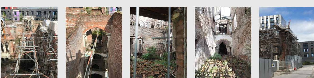
Current building condition
