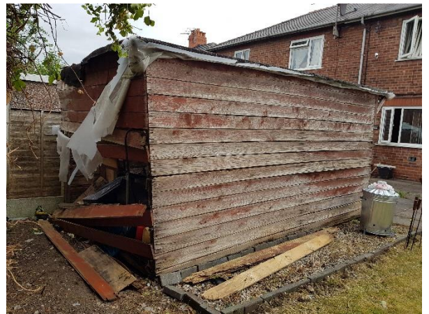
Existing rear outbuilding
