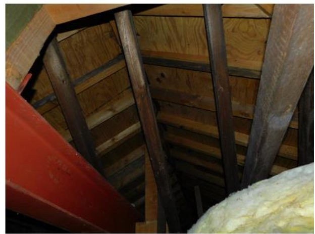
PHOTO 10 Underside of Main Roof
