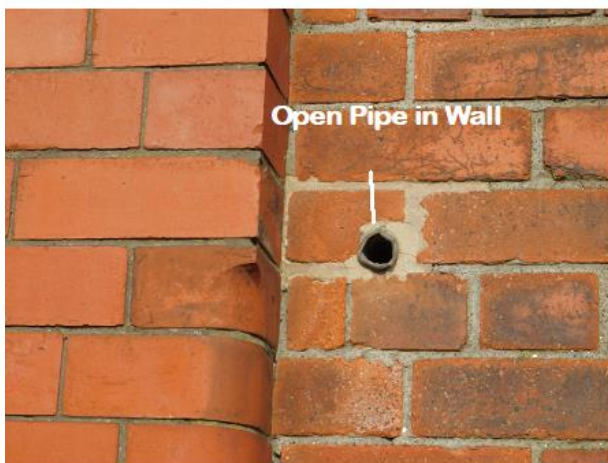
PHOTO 9 Part of Eastern Elevation
