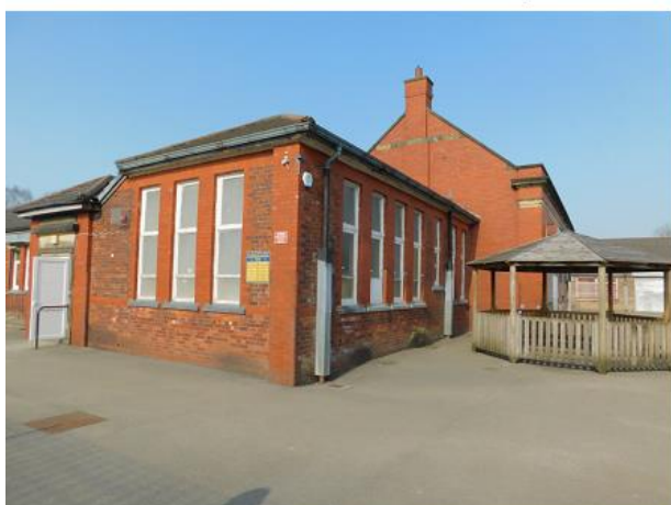
PHOTO 3 North-eastern Corner of Complex
