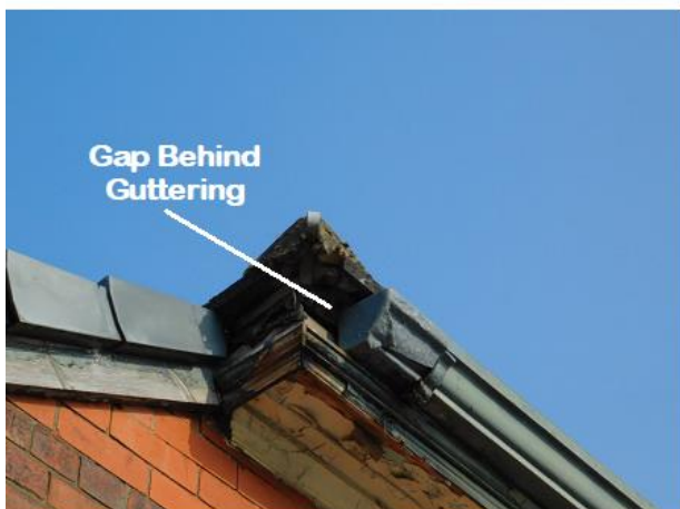
PHOTO 5 South-eastern Corner of Main Roof
