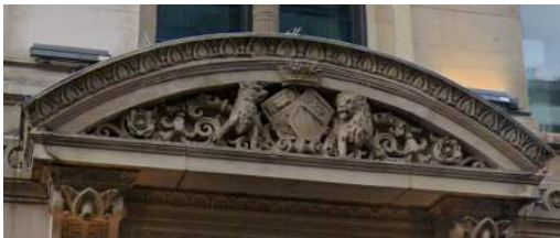
Entrance canopy ornamental pediment detail
