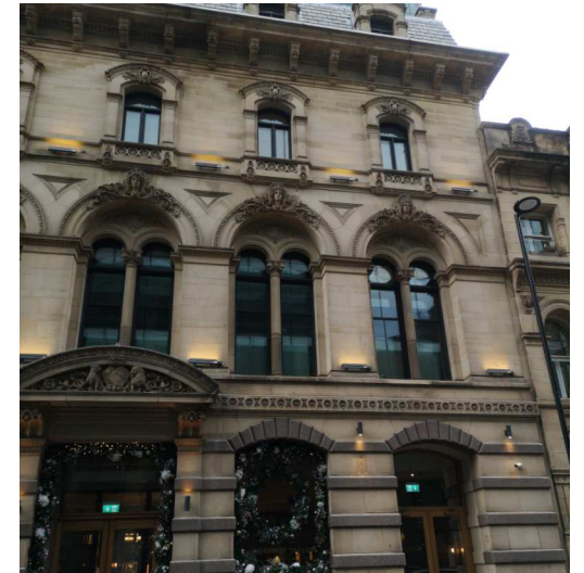
Existing Facade Lighting - Booth Street Facade
