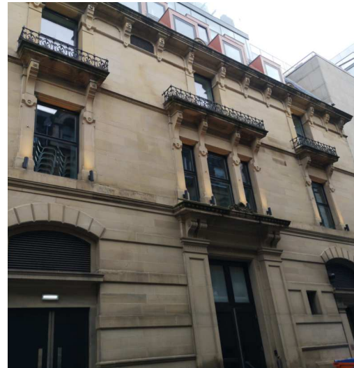
Existing Facade Lighting - Kennedy Street Facade
