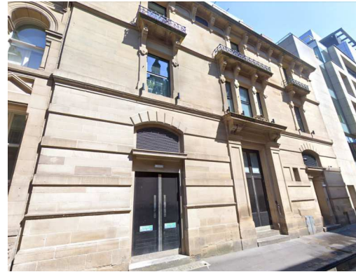
Street View - Kennedy Street Facade
