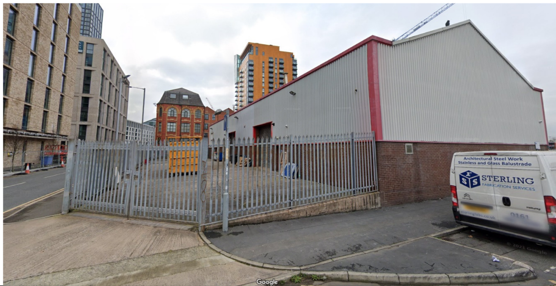
View from Addington Street / Cross Keys Street to show vehicle access gates
