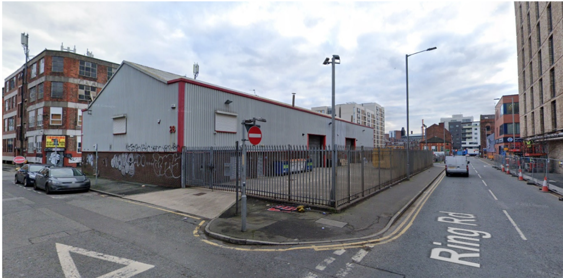
Mason Street Junction where it joins the A665 ring Road Addington Street Vehicle access gates in the centre of the image
