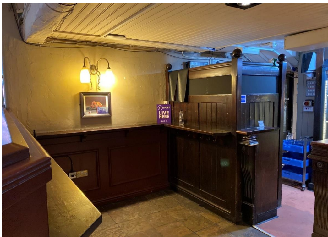
Figure 4.12: General image showing the glass wash area of the main bar with modern timber panelling, 19 th century beam and modern timber panelled ceiling (2021)
