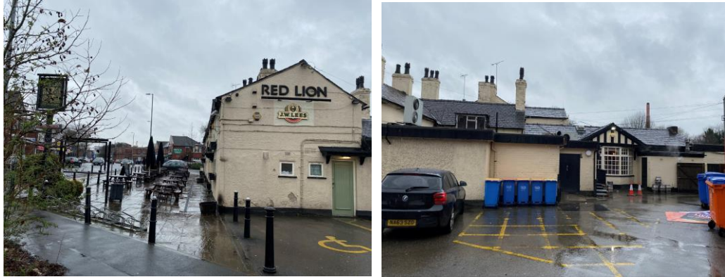
Figure 4.2: The Red Lion today, looking south from Marriot Street, showing the northern elevation of the building. The various later extensions to the rear of the building are visible in the right-hand image
