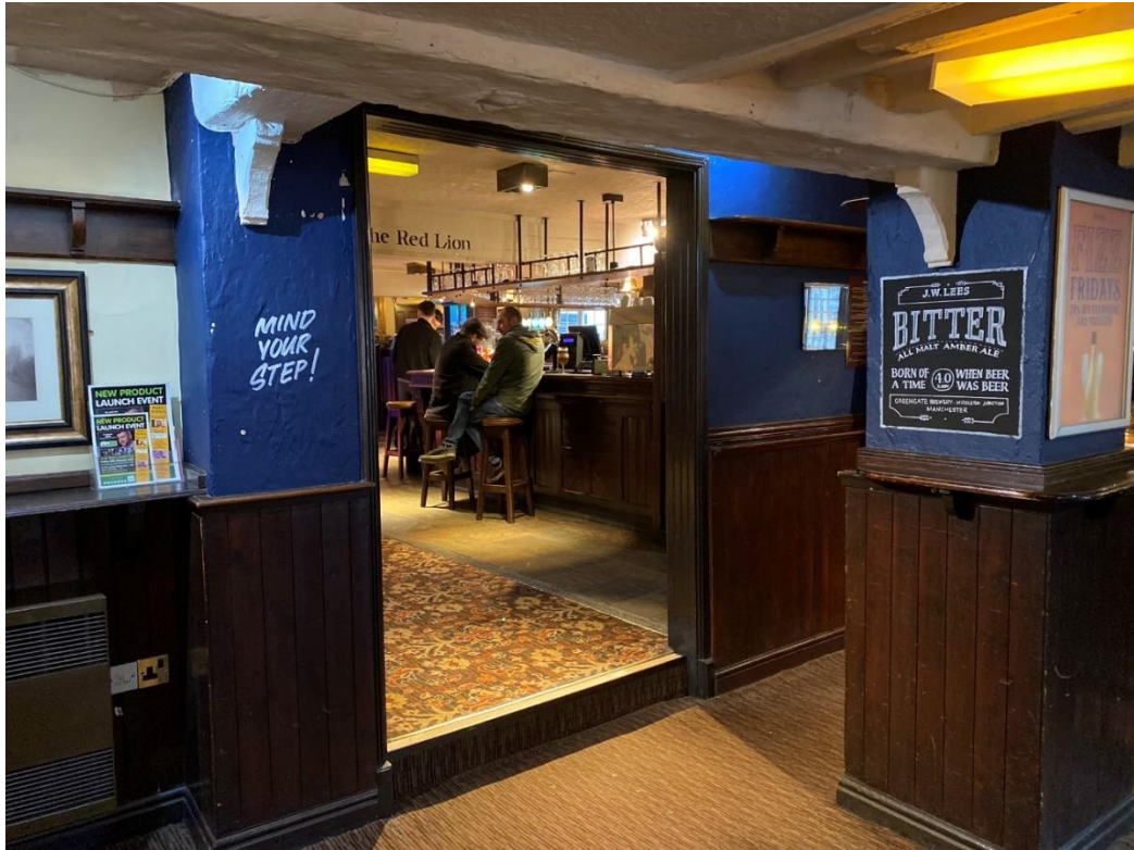
Figure 4.8: General image looking through from the front part of the building (at the east of the building) through to the bar. The 17 th century beams are visible in this image along with some surviving brackets (2021)
