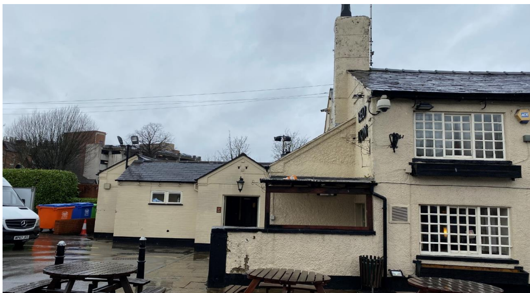
Figure 3.14: The southern end of the Red Lion building, looking west and showing the modern additions at the southern end of the building (2021)
