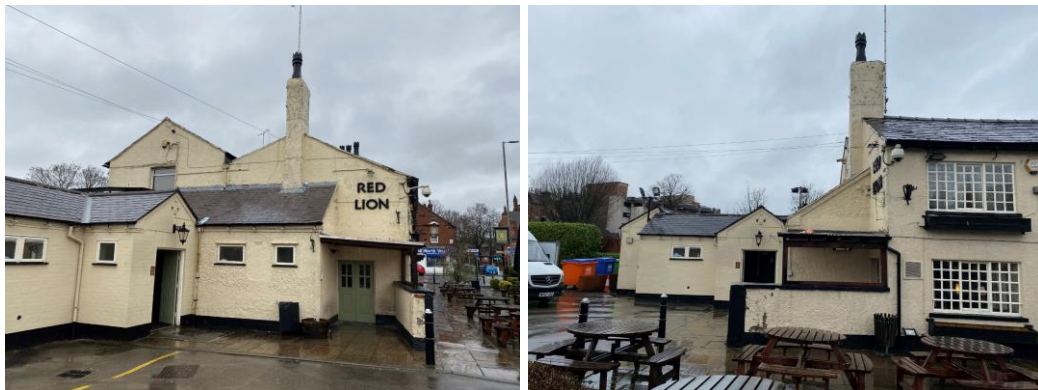
Figure 4.3: The Red Lion today, looking north, and showing the modern additions to the southern elevation of the building.
