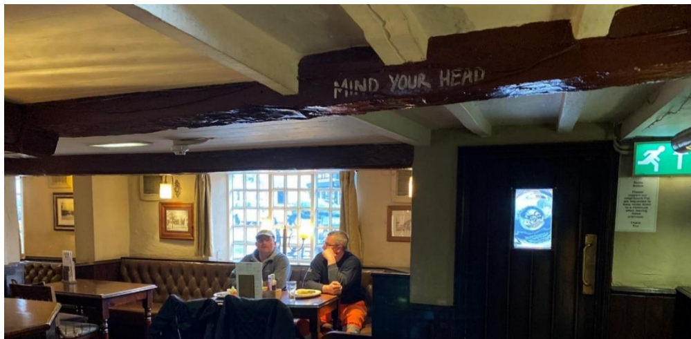
Figure 4.7: Front bar area showing the existing modern fixed seating. The low ceilings and visible historic beams of the building are visible in this image (2021)
