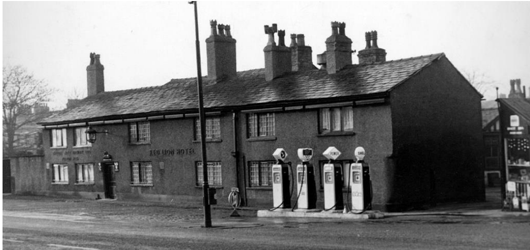
Figure 3.11: 1959 Photograph showing the Red Lion (looking south-west). A set of petrol pumps are shown in front of the pub and an associated kiosk building is visible at the right hand edge of the image. (Manchester Local Image Collection)
