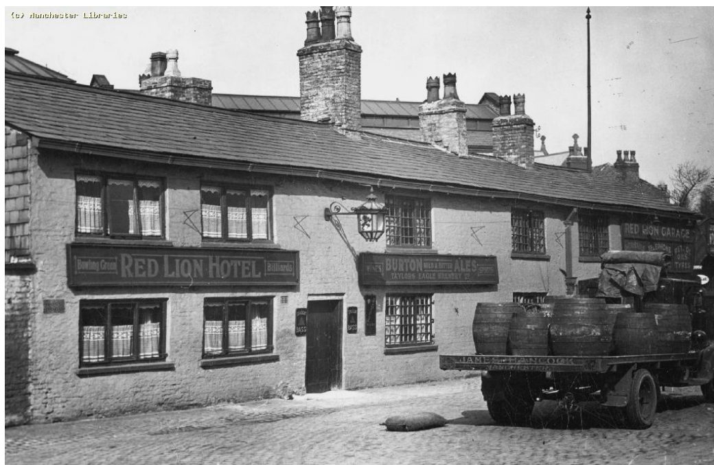
Figure 3.7: The Red Lion in 1932. Signage on the building indicates that the northern end of the building was in use as the Red Lion Garage by this date. (Manchester Local Image Collection)
