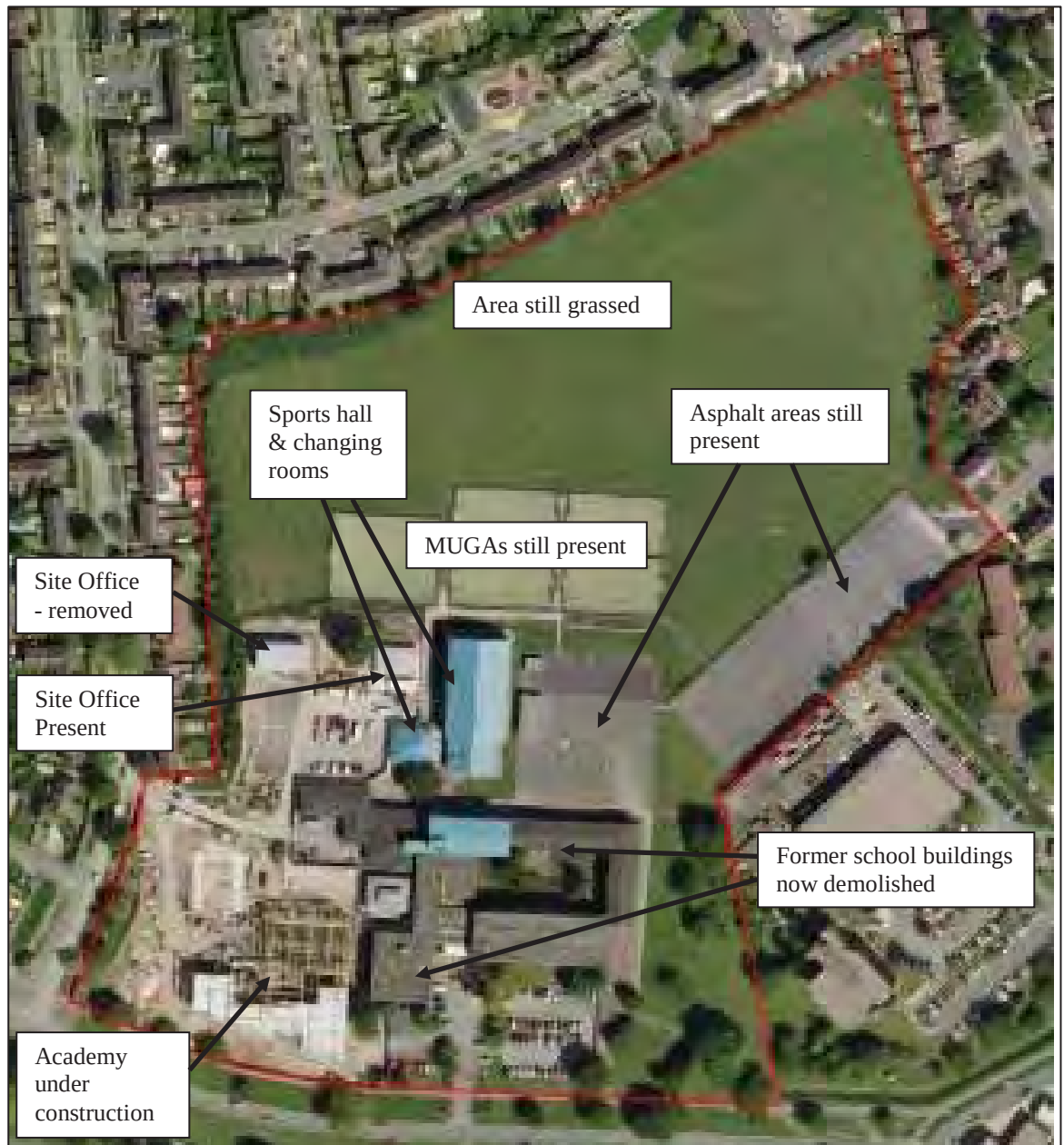
Figure 2: Aerial Photograph from 02/06/09 When the Academy was Under Construction (from Groundsure report, Appendix D)
