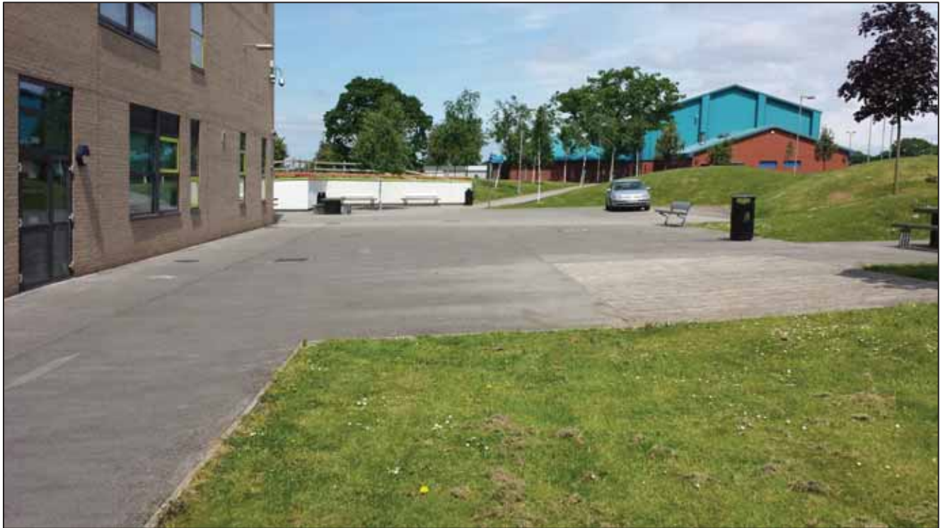
Photograph 1: Northerly View of Northern Area of New Building
