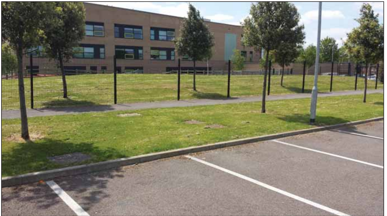
Photograph 9: South Westerly View of Northern End of Existing Main Academy Building
