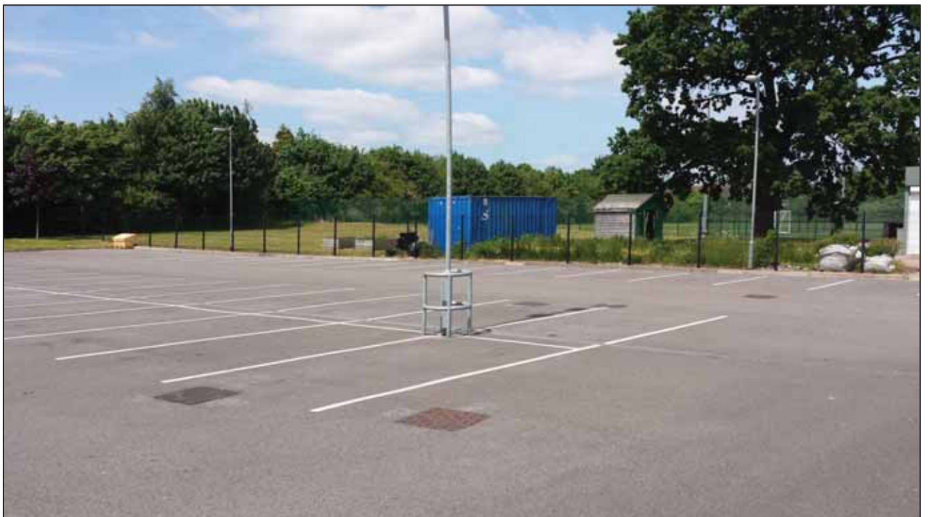
Photograph 10: North Westerly View of Northern Car Park
