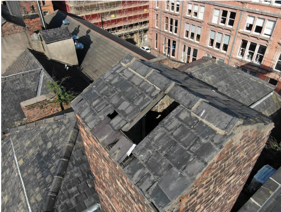
Figure 4 – Image from drone survey showing the existing lift shaft to be removed in the foreground.
