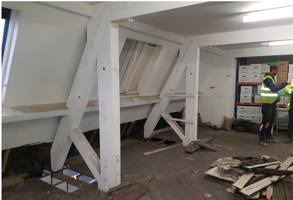
Figure 2: Photograph of internal roof space to 47 Dale Street
