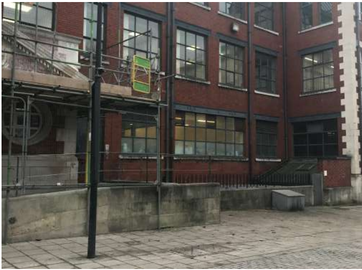
Bridgeford Street Elevation, ramp to museum staff entrance and basement access to the Sub-station.
