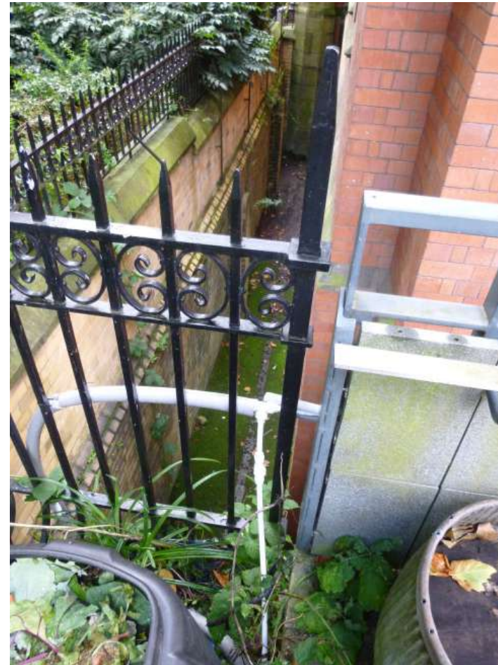
Historic Cast Iron Railings at Rutherford Building
