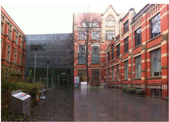
Stitched photograph of the site, looking north-west from Coupland Street, showing its full width.
