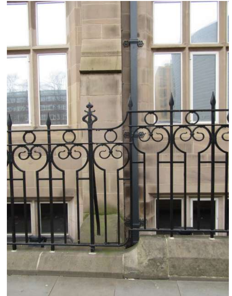
Railings on Oxford Road. Although historic in character, these are modern railings with modern fixings.
