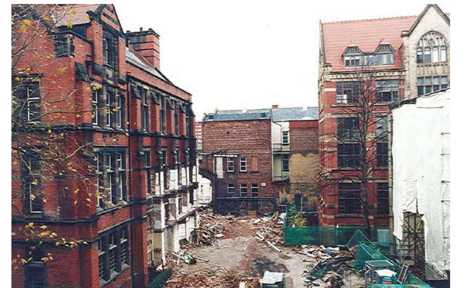
Museum Courtyard post demolition
