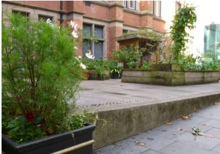
The current ramp provides a level access to the museum entrance, addressing the 1.1m level change.
