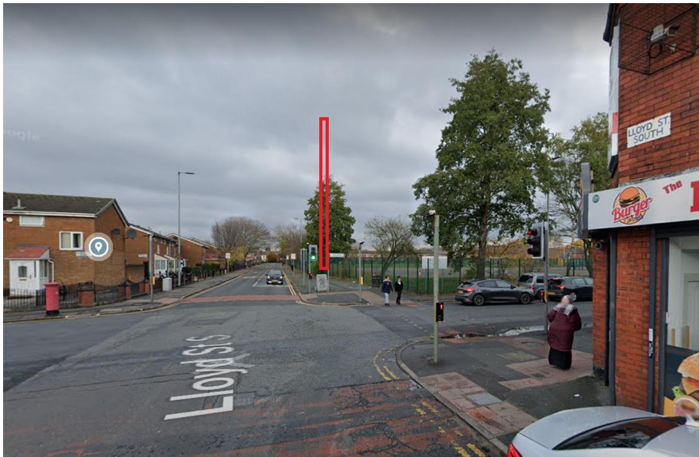
View north on Lloyd Street towards the proposed mast siting
