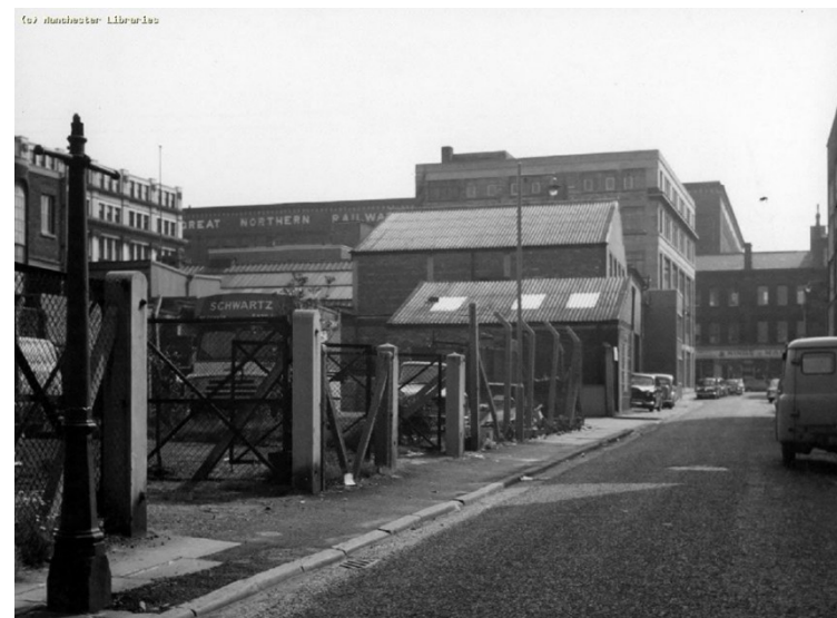
Plate 11: Camp Street, 1964 after demolition.
