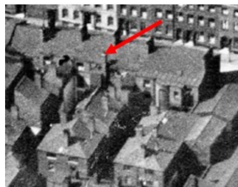
Plate 24: The chimney at No.15 in 1930.
