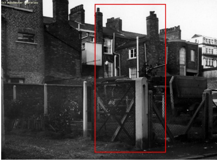
Plate 12: Rear of No.13 from Camp Street, 1964 after demolition.
