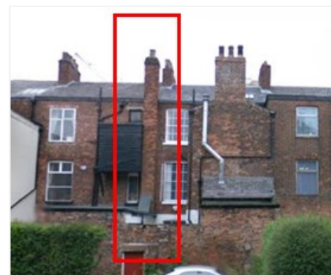
Plate 23: The chimney at No.15 in 2008.
