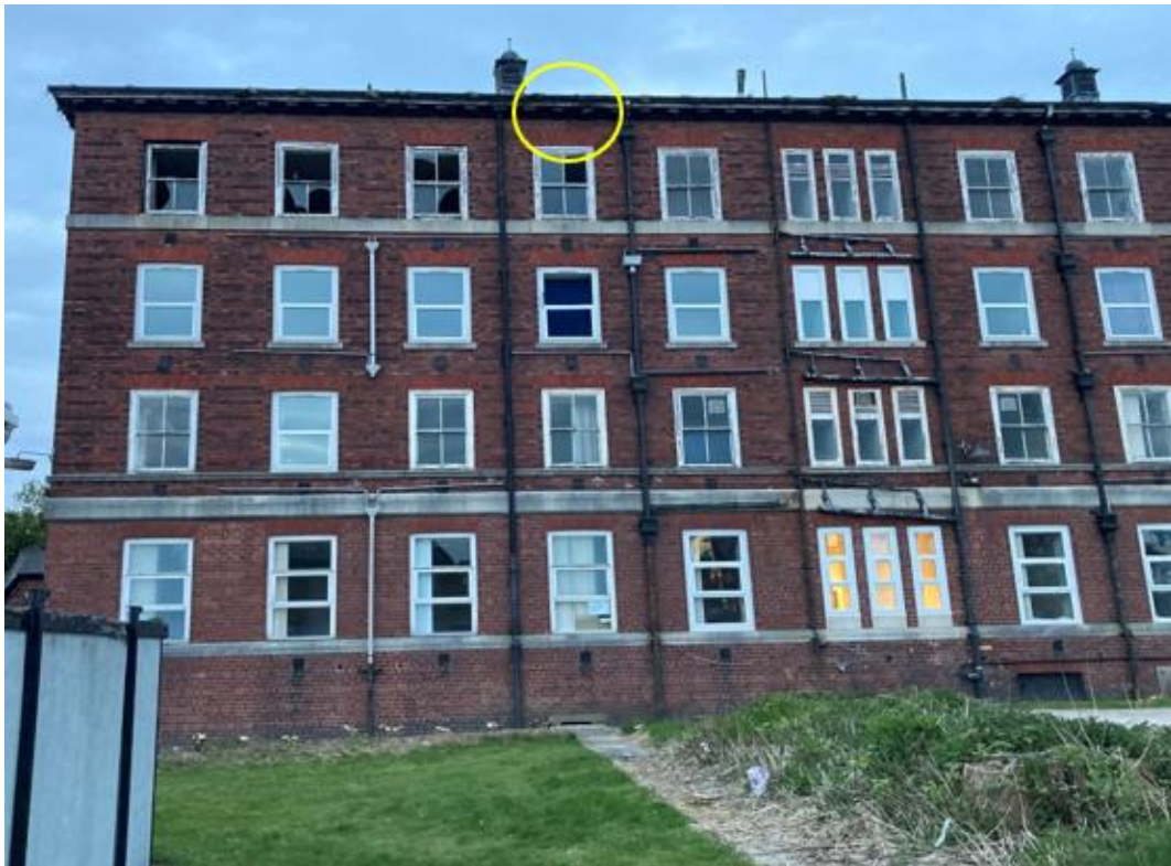
Plate 1. Location on eaves where single common pipistrelle emerged at 20:41.
