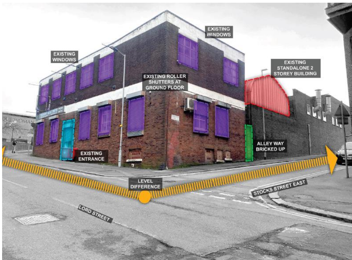
Figure 9: Lord Street/ Stocks Street East Alterations
