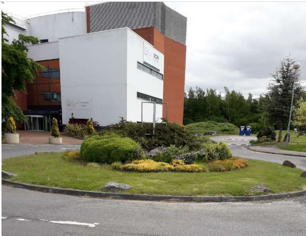
PLATE 1 CENTRAL BUILDING AND ROUNDABOUT
