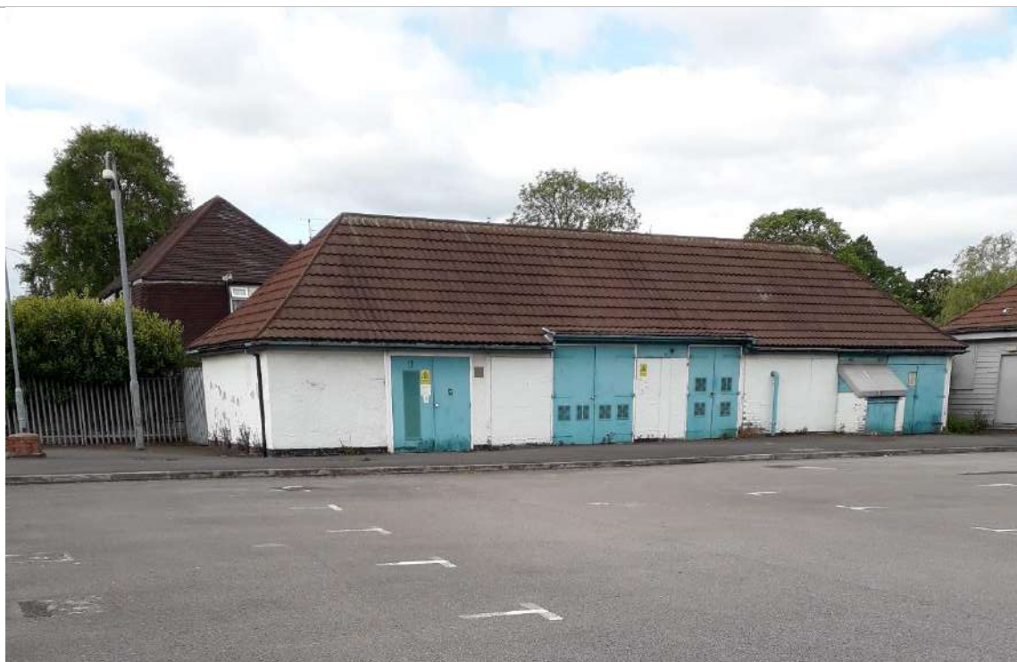
PLATE 2 ELECTRICITY SUBSTATION BUILDING ON WESTERN BOUNDARY OF SITE
