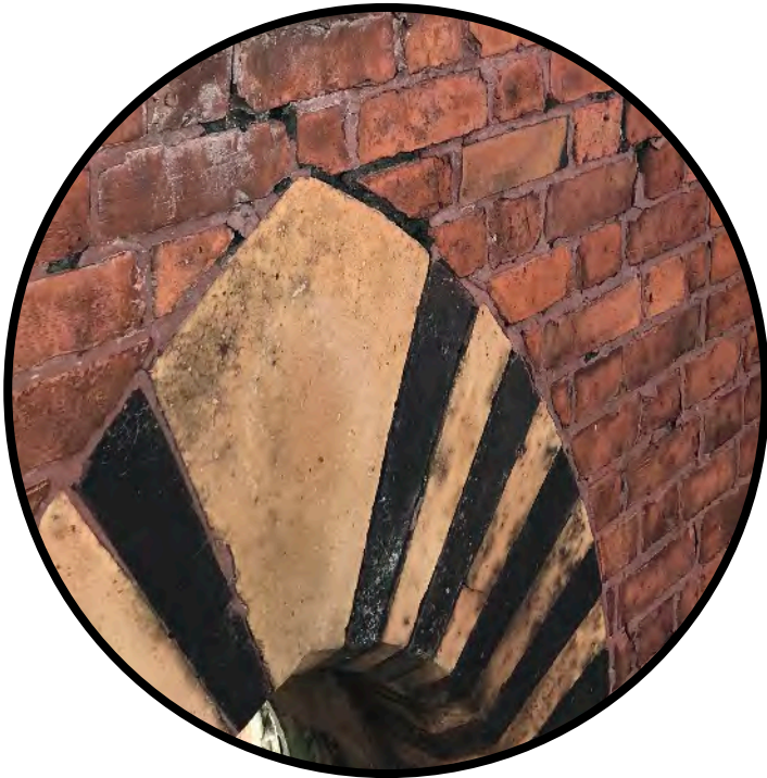
Arched Lintels to match existing
