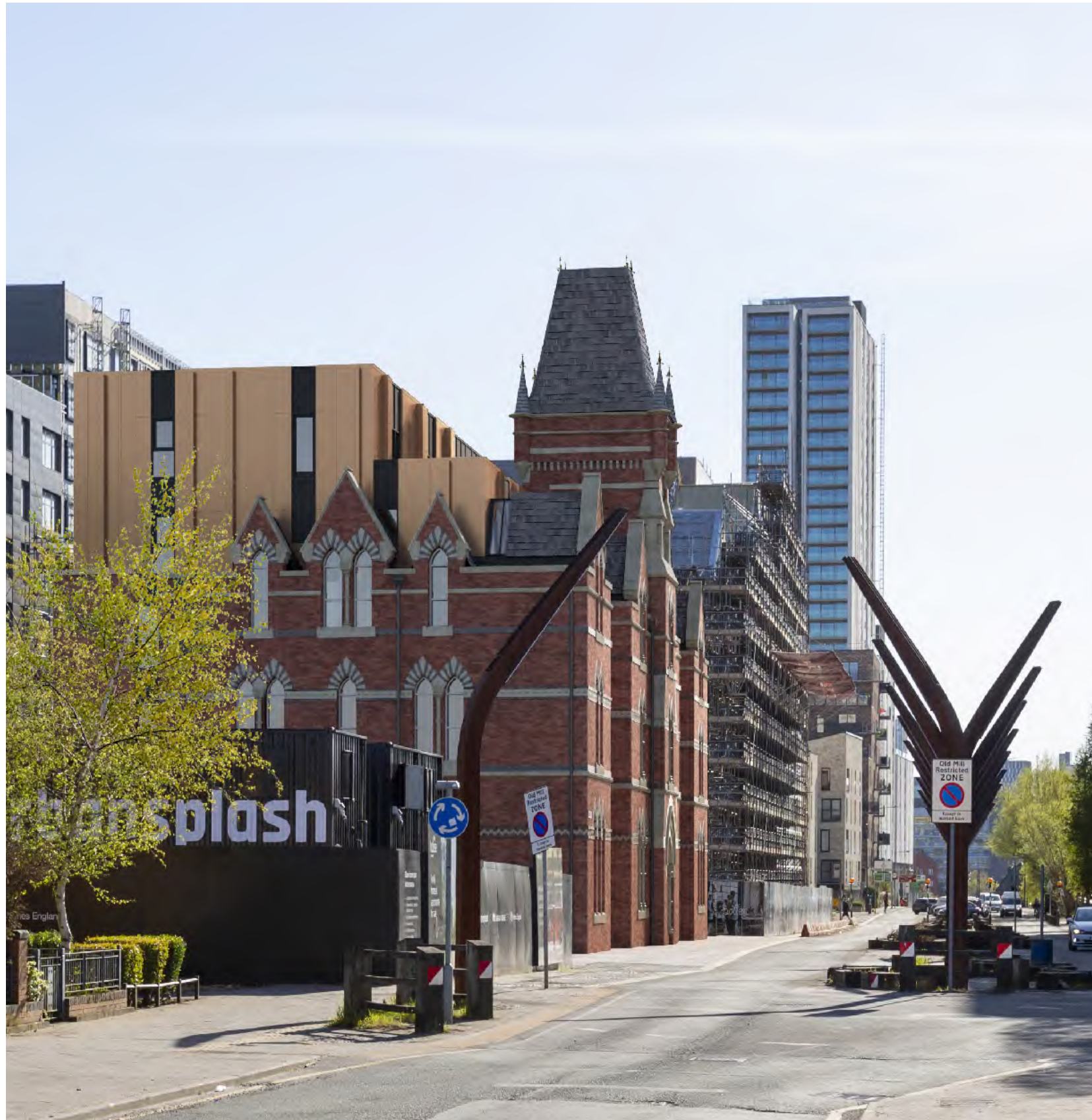
View looking at North East Elevation from Old Mill Street
