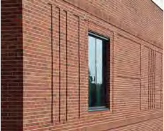
Image showing recessed brickwork
