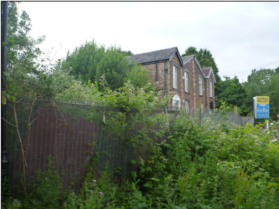
Appendix 2.2: View across the site along Park Grove, looking west from the entrance to the railway underpass
