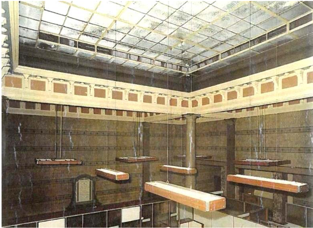
Figure 8: A similar view taken after the building was sold for redevelopment in the 1980s, showing the exposed original terracotta clad walls and pink granite columns supporting the raised glazed roof (now all removed).
