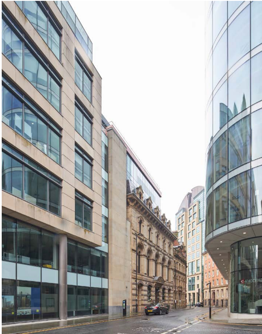
Figure 36: A view looking west along Booth Street towards the principal elevation of the King Street Townhouse, illustrating the largely modern and medium-rise nature of buildings in this part of the Upper King Street Conservation Area.
