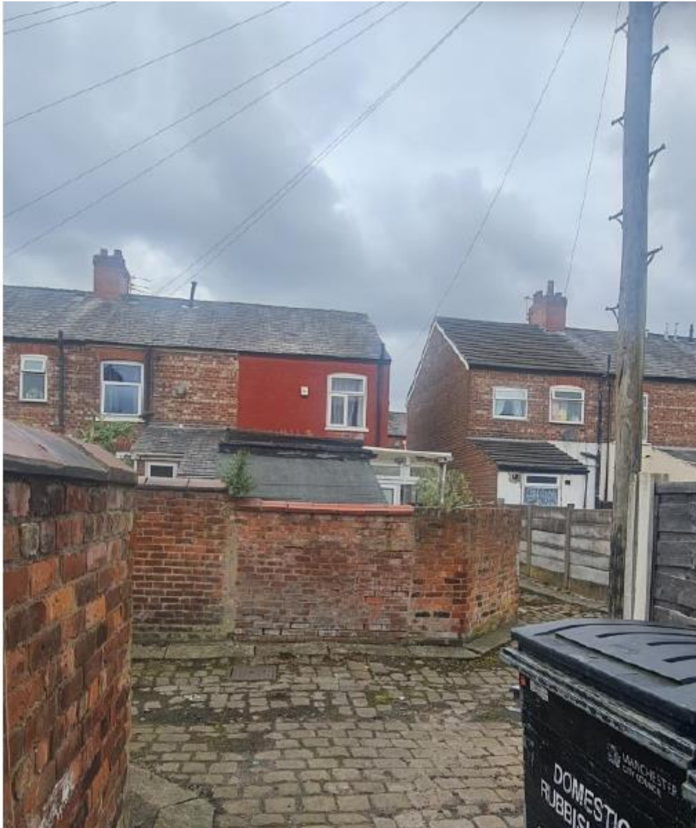
Fig. 1 – Rear of the application site
