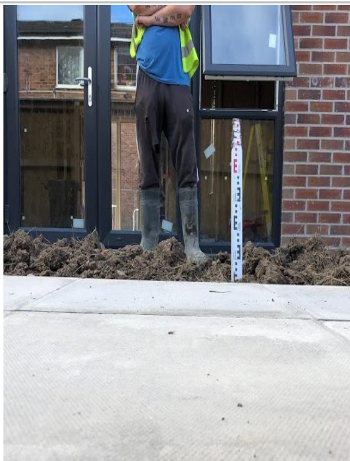
Depth of Cover System at Ground Level
