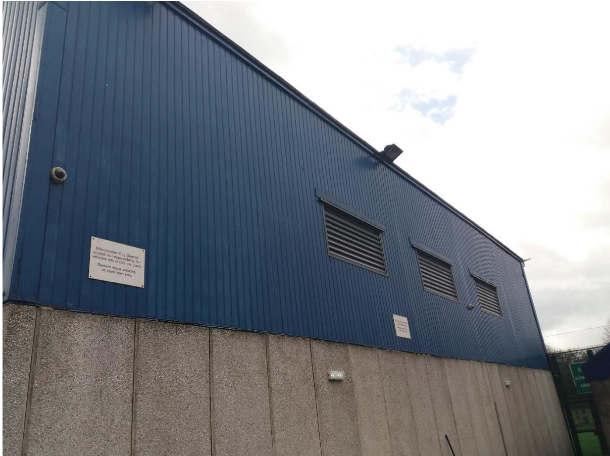
Photo 5: High level profiled timber cladding at elevation number 3.
