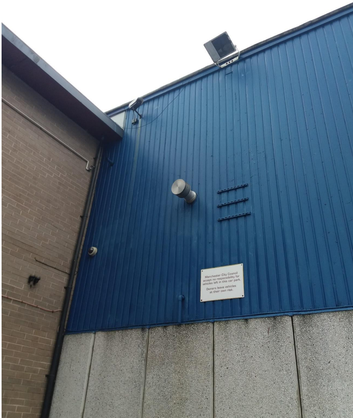
Photo 6: High level profiled timber cladding at elevation number 4 at abutment to brick elevation
