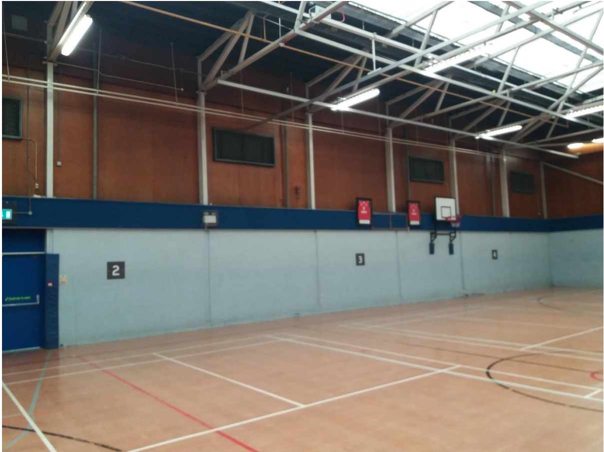
Photo 7: Internal view of the sports hall, showing the steel frame and roof structure.
