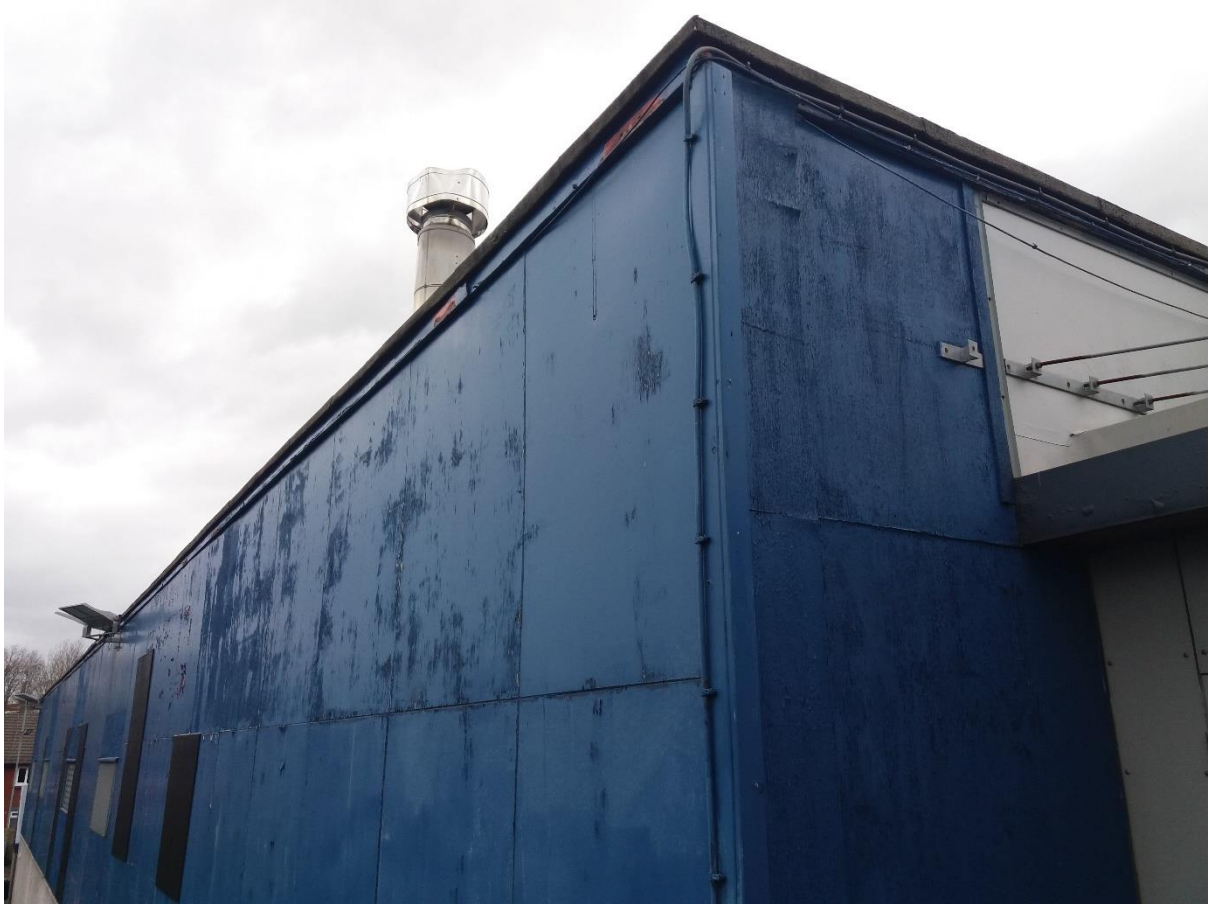
Photo 4: High level flat timber cladding at elevation number 2 at junction with first floor fire escape stairs.
