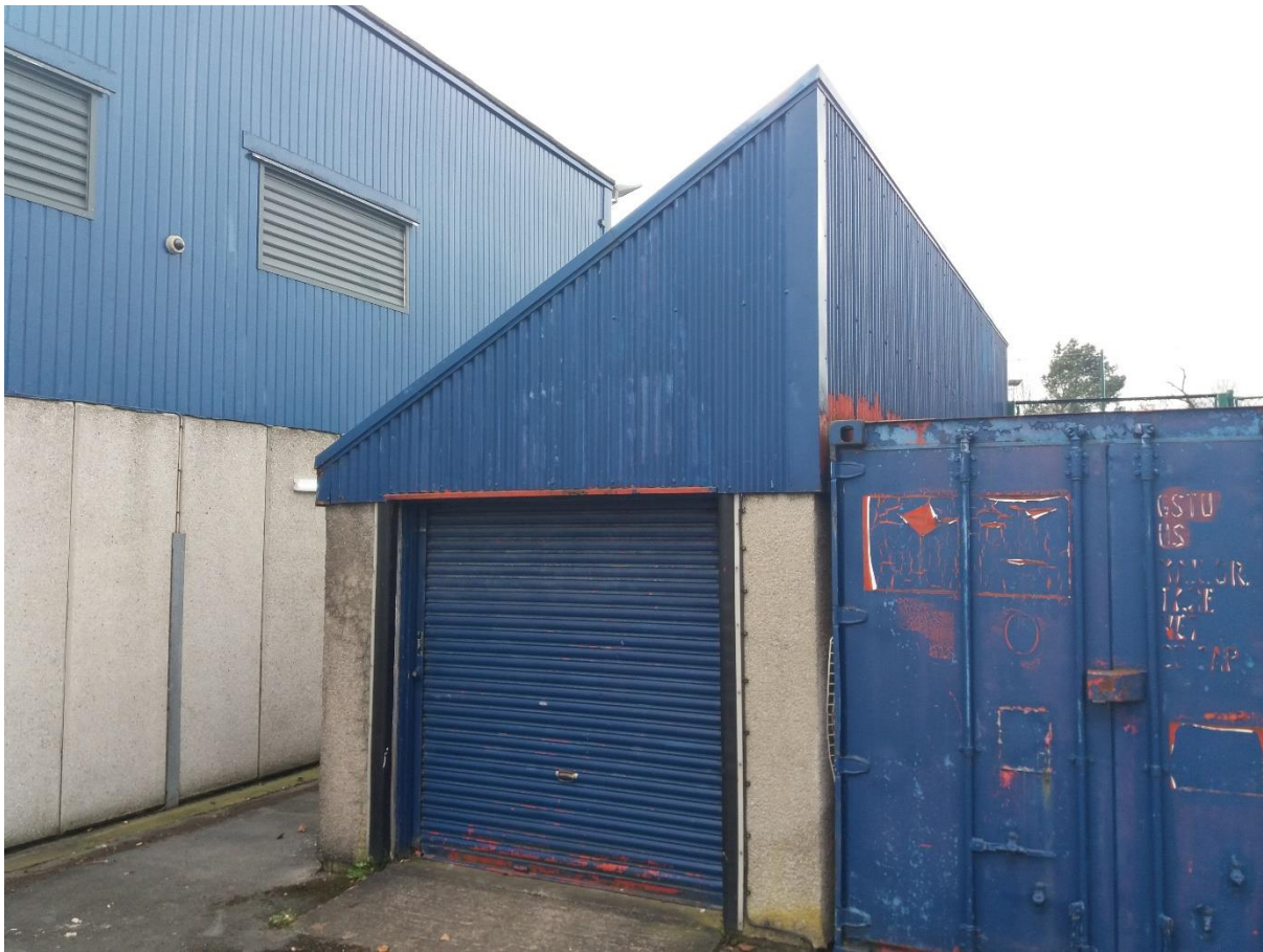
Photo 11: Garage Outbuilding located adjacent to elevation number 3.
