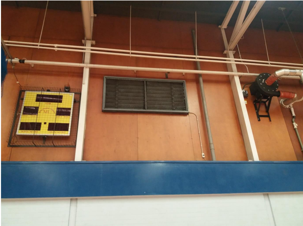
Photo 8: Internal view of the high-level ventilation louver to the external wall of the sports hall.
