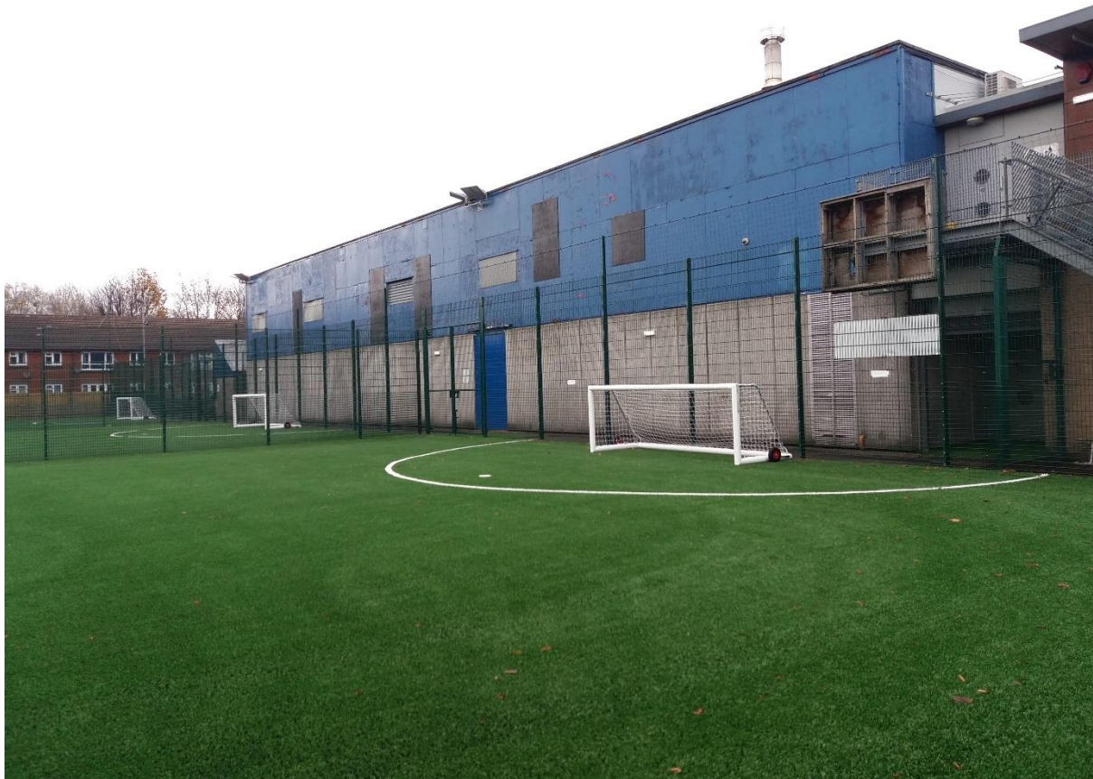
Photo 3: Existing blue coloured high-level timber cladding and low-level concrete cladding panel to the external elevation facing the football pitches. Elevation number 2 on drawing reference ALC-MCC-B01-XX-DR-A-0013.
