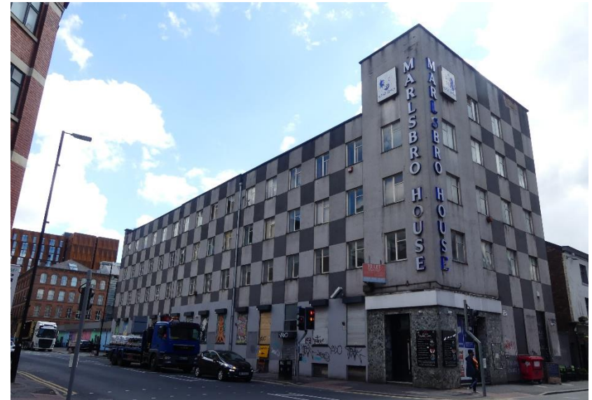
Figure 4.1: Marlsbro House, Newton Street
