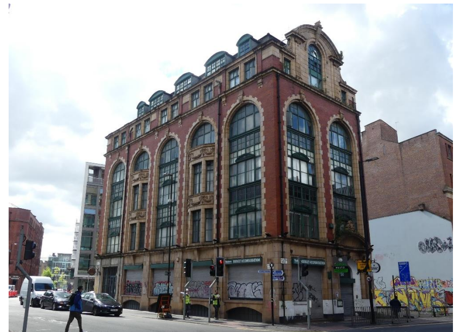
Figure 4.3: Newton Buildings, Hilton Street Elevation
