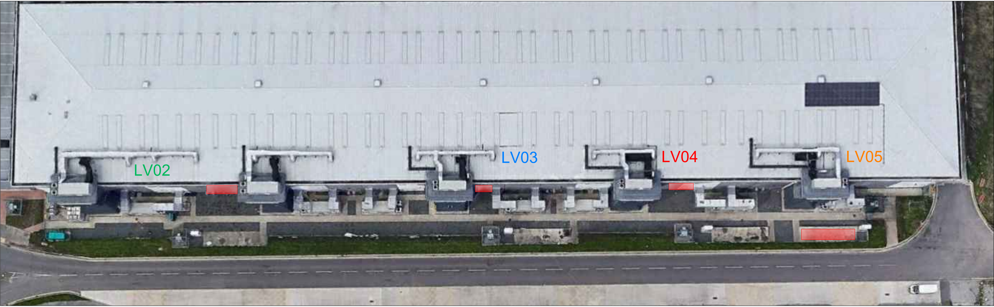
AERIAL IMAGE OF INVERTER LOCATIONS
