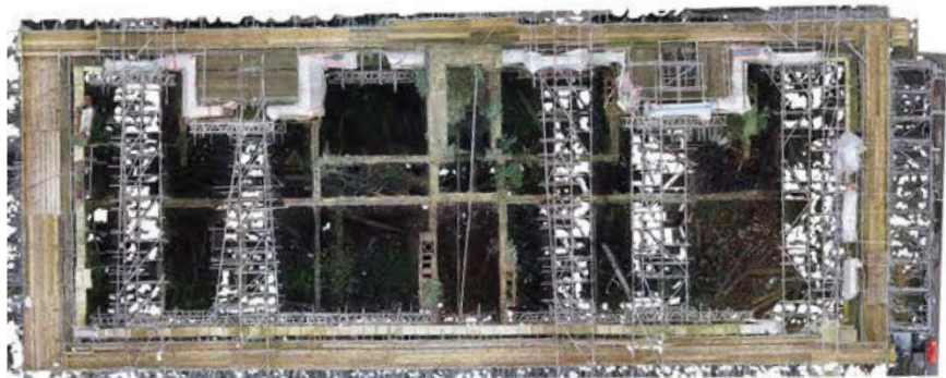
Figure 16: Aerial view of the interior showing remaining interior walls
