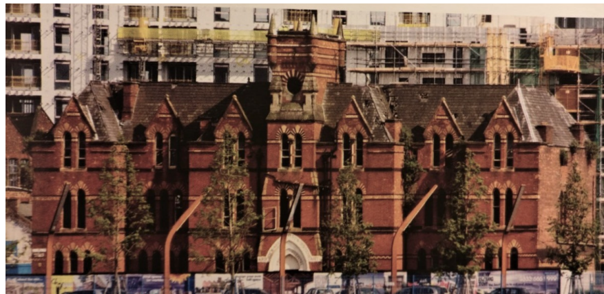
Figure 10: Main elevation showing the roofscape before destruction by fire
