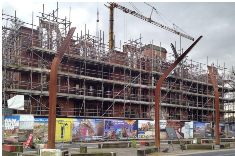
Figure 17: Present condition, Old Mill Street elevation, 2020
