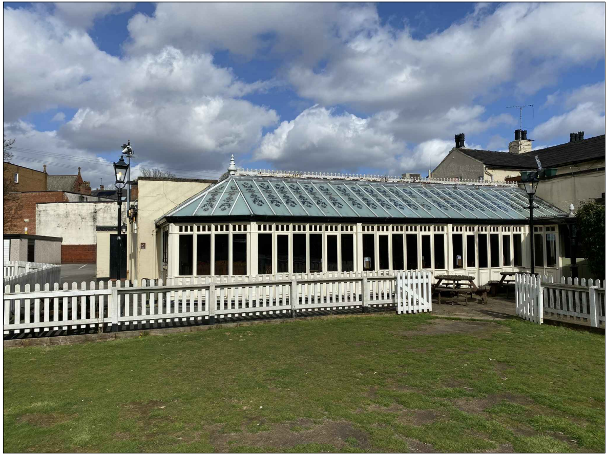
SOUTH ELEVATION PHOTOGRAPH
