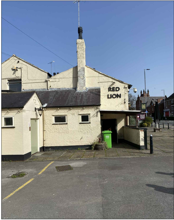
SOUTH ELEVATION PHOTOGRAPH
