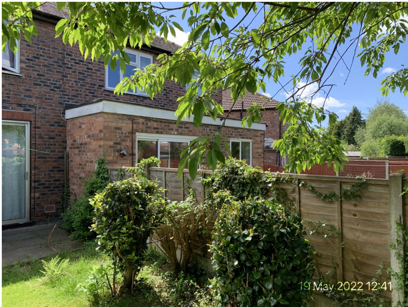
Photograph 2 No. 12 Broughville Drive extension as viewed from the application site. Source Case Officer Site Photograph
