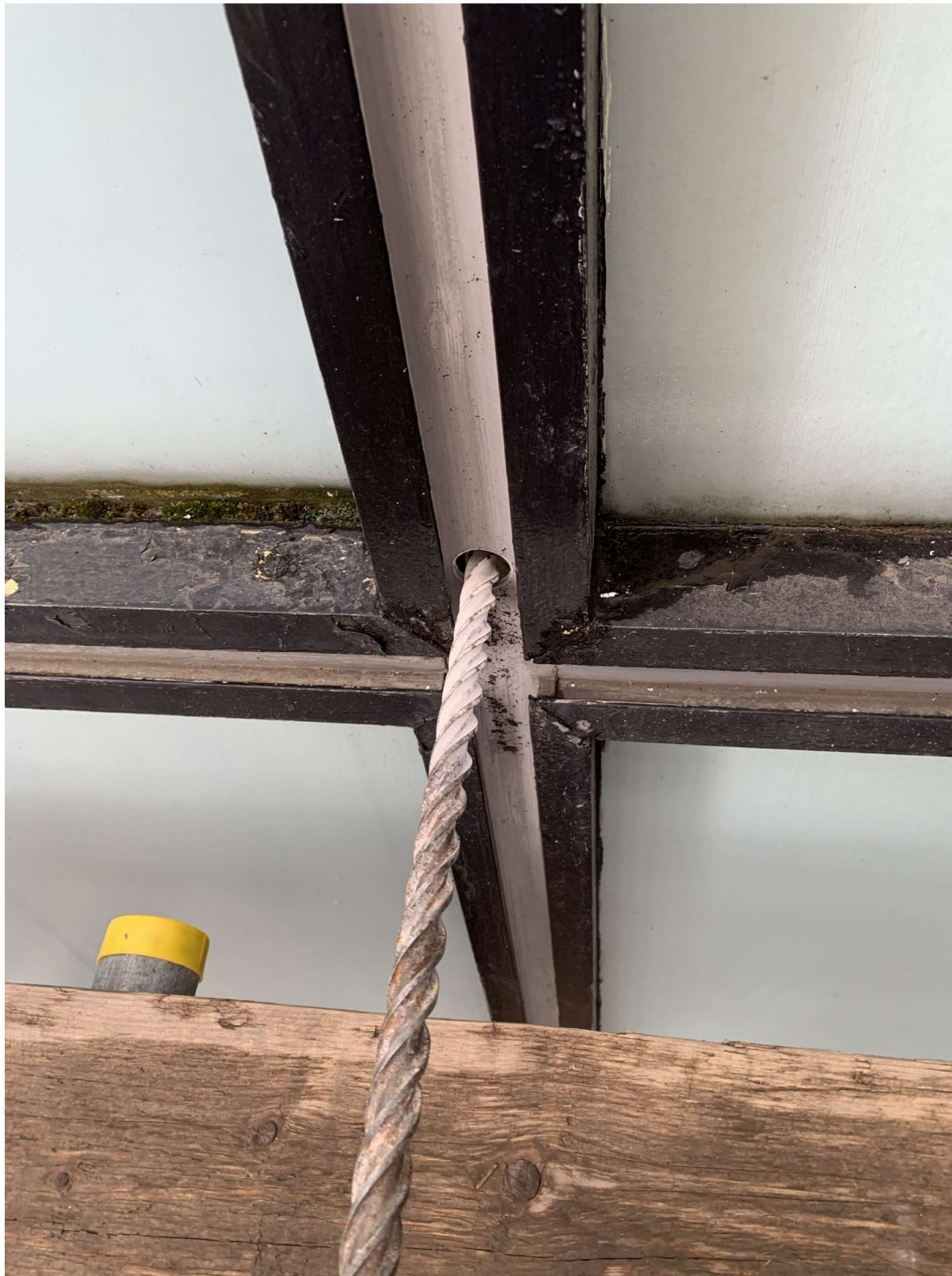
5. 120mm hole drilled through masonry.
