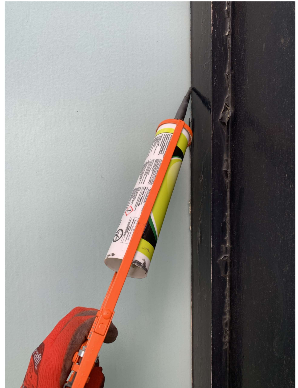
11. Structural mastic to be installed to the perimeter of all windows
