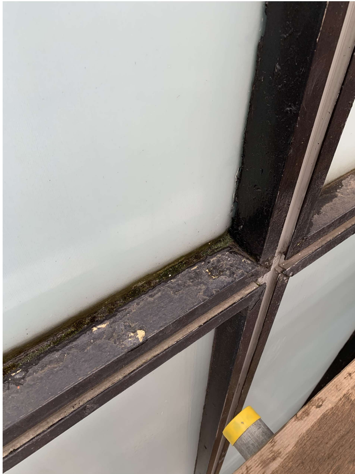
10. Windows and frames to be cleaned - Soap and clean water only
