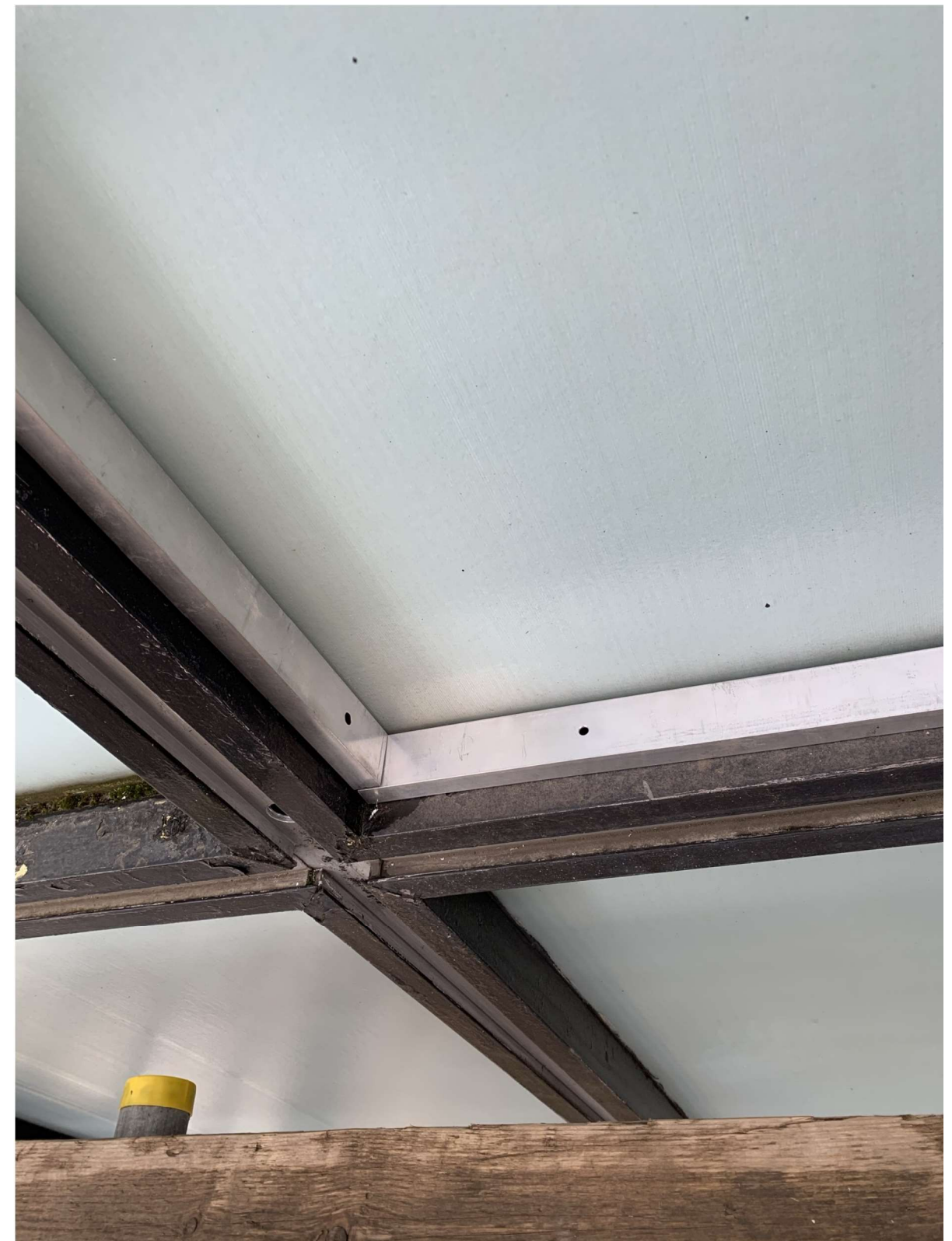
13. Aluminium beads PCC Black to be installed to all 4no sides the 199 windows. These will be notched around the angles
