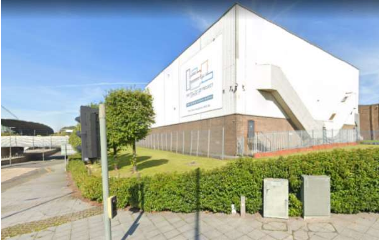
Sharp Project from Oldham Road looking north
