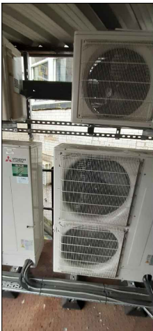
Existing Condenser Location
