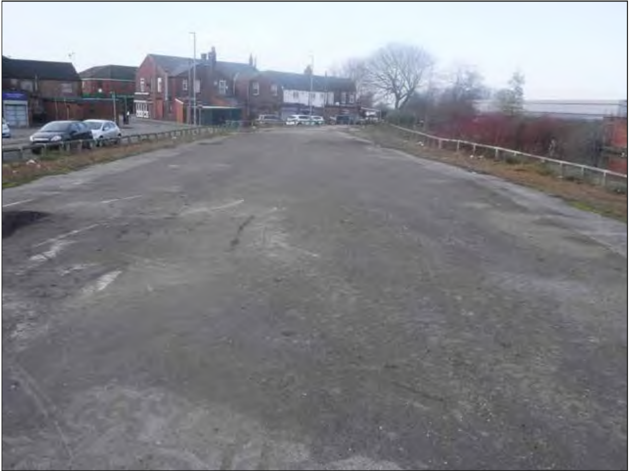
Plate 35. SW view of Area C from centre
