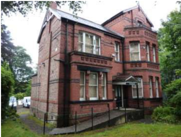
West and North Elevations of the building showing rampway access to the front entrance.
