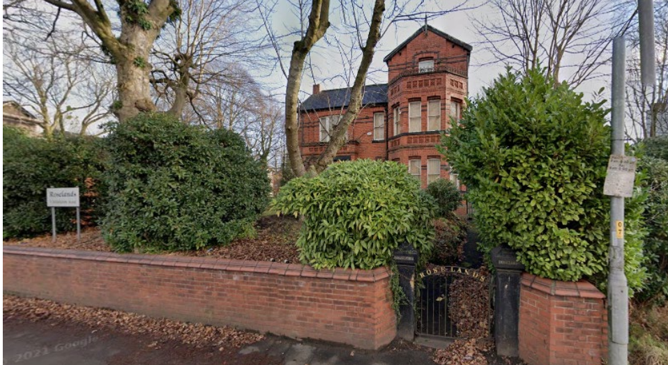
Existing Pedestrian access point from Middleton Road.
