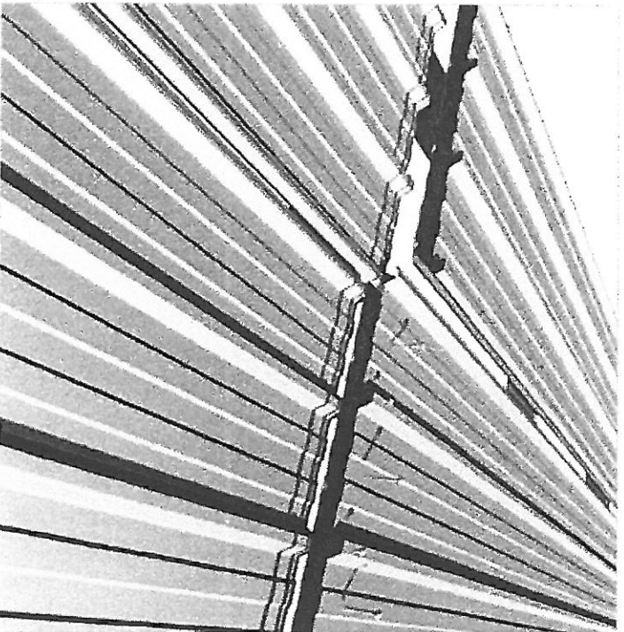
Figure 1: Roof panel - end and lap fixing
