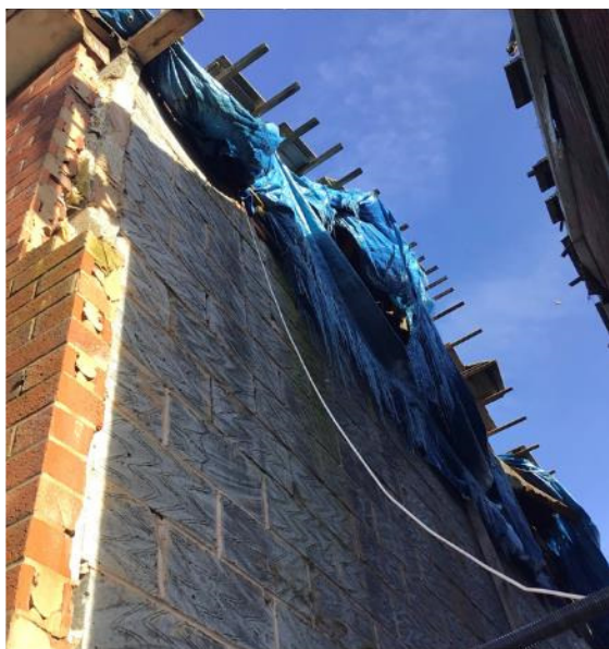
South aspect. Bat roost potential present with gaps in wall cavities and gaps under roof tiles.
