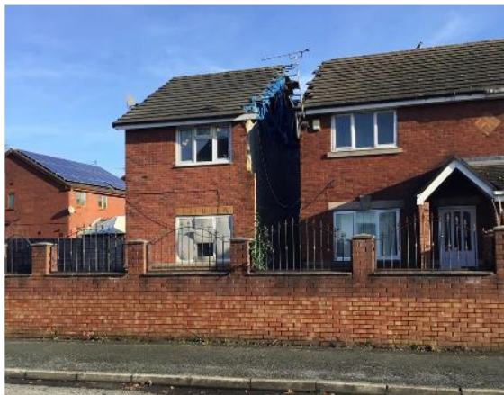
View of western aspect of partly demolished property (within red line boundary) and property to the immediate south.
