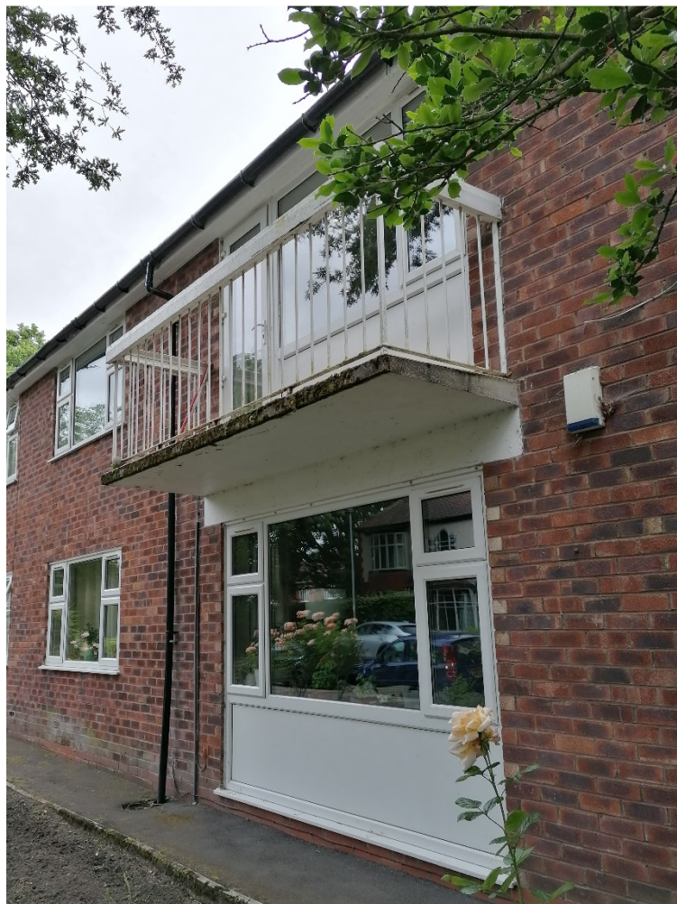
Fig 5: View of balcony on the Northeast Elevation, Holmwood Road.
