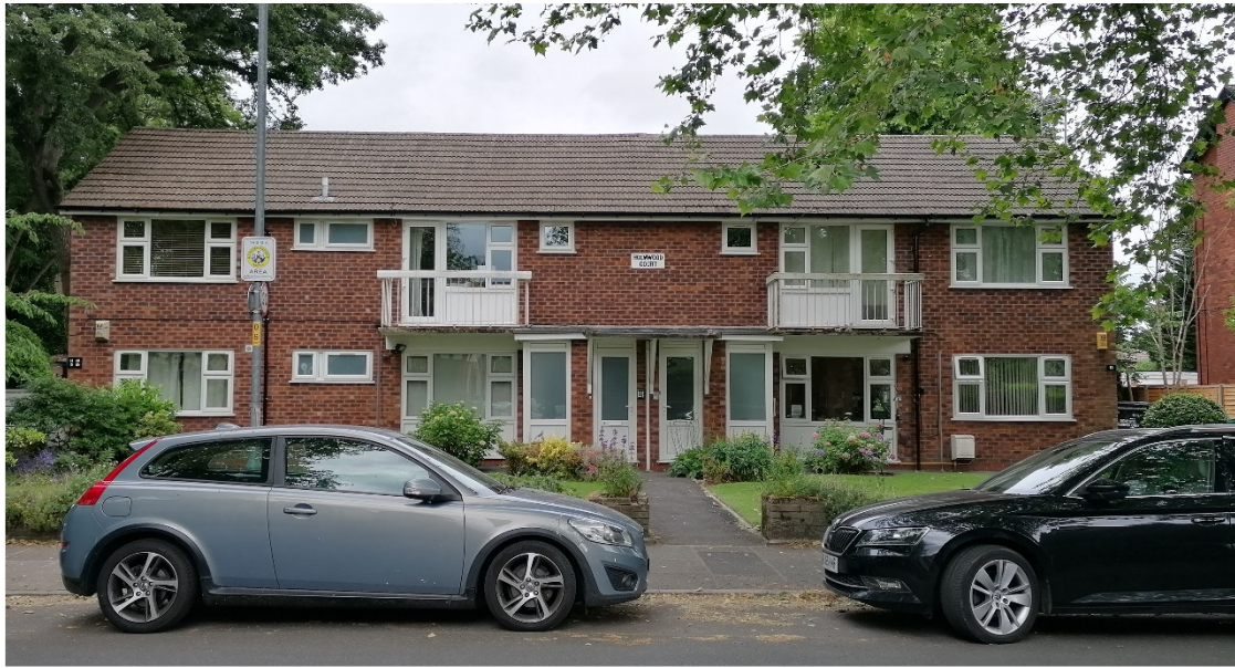
Fig 2: Southwest Elevation, Ballbrook Avenue.
