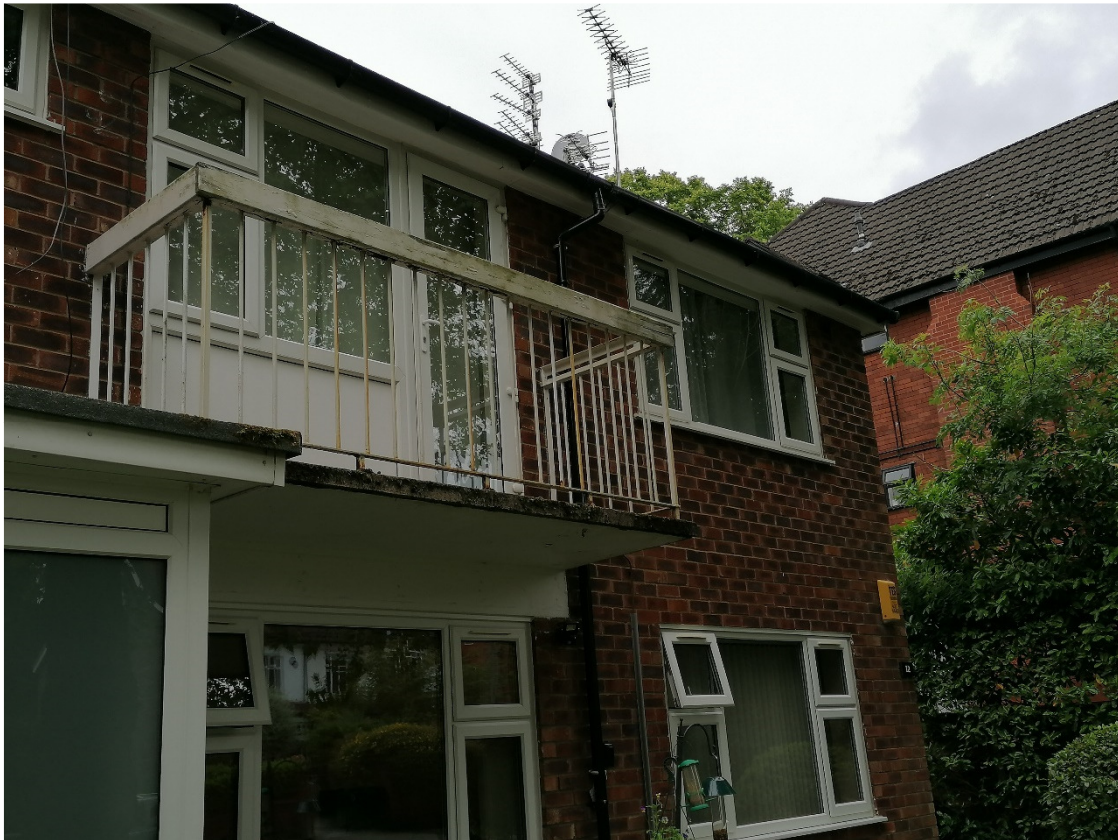
Fig 3: View of existing steel bar and timber rail balustrades, Ballbrook Avenue.
