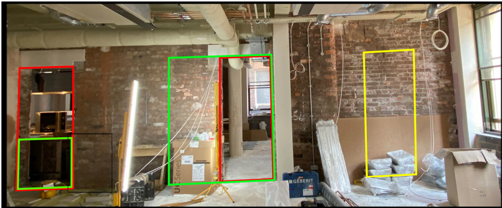
EXISTING ORIGINAL WALL ON GL 6
