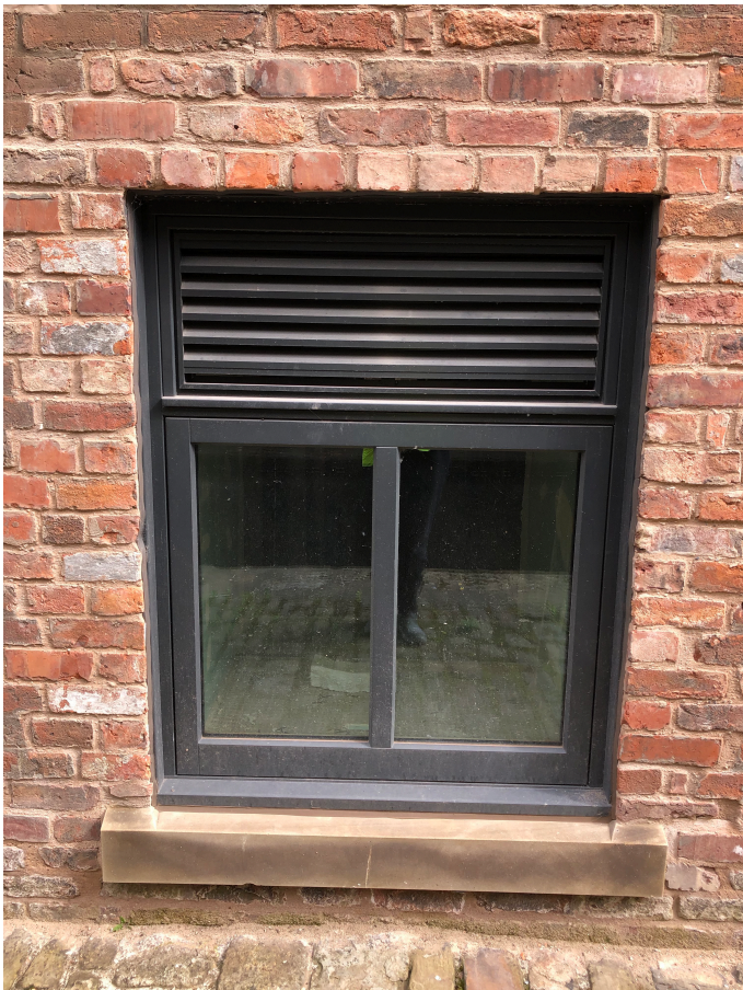
example of making good/brick infill to new aperture (minto - canal st)
