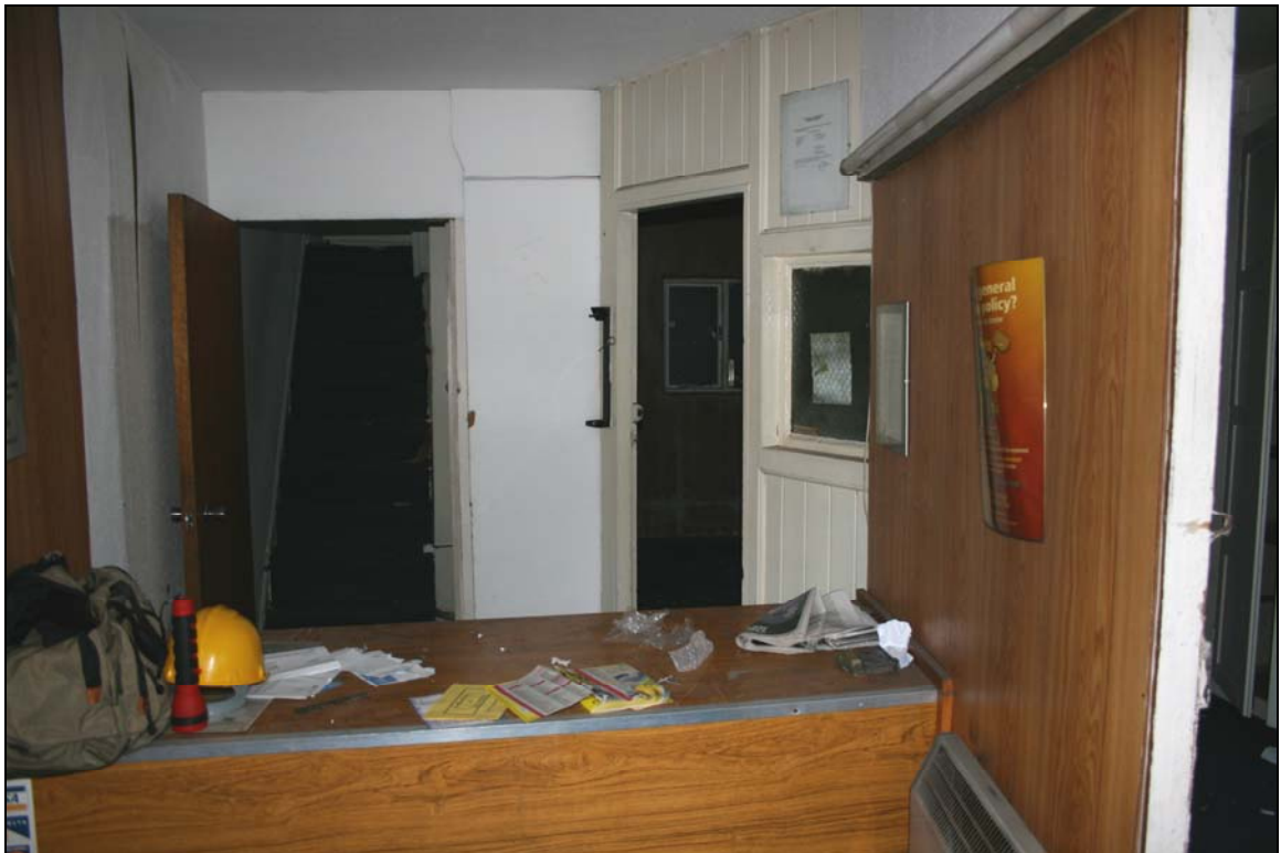
19. Modern reception area, with staircase beyond and doors to main room on right
