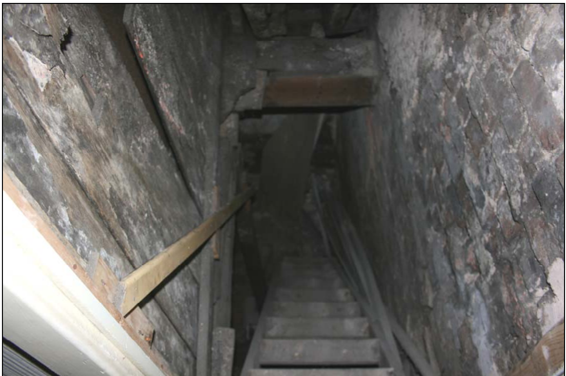
33. Arch formed by converging flues on second floor
