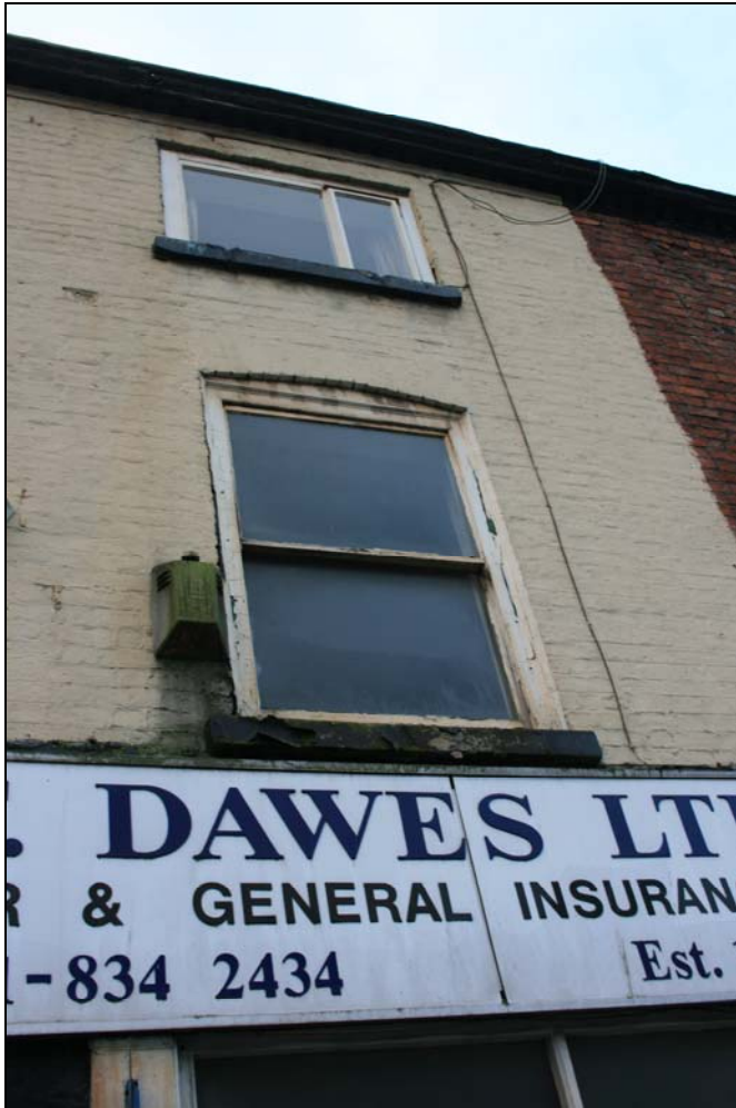
15. First and second floor windows
