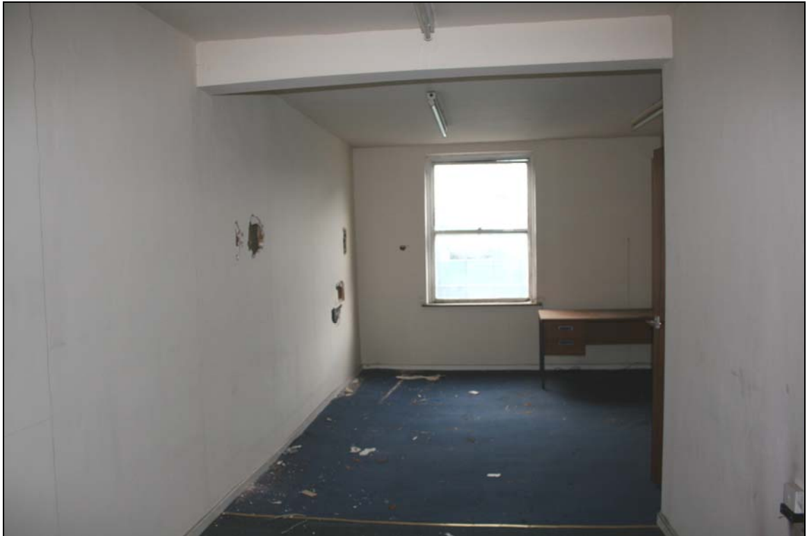
29. Looking to front of building on first floor
