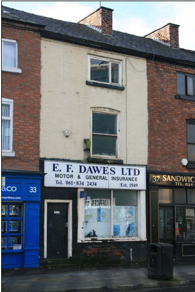
6. Main elevation of the property to Liverpool Road
