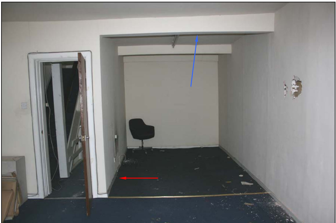
28. Front first floor room looking to rear, showing original line of crosswall (blue arrow) and site of former door from landing to rear room (red arrow)
