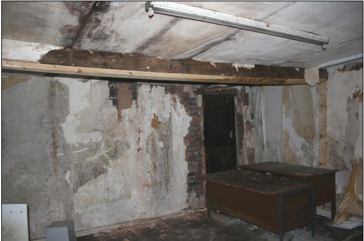
25. Interior of rear extension, with external door to passage
