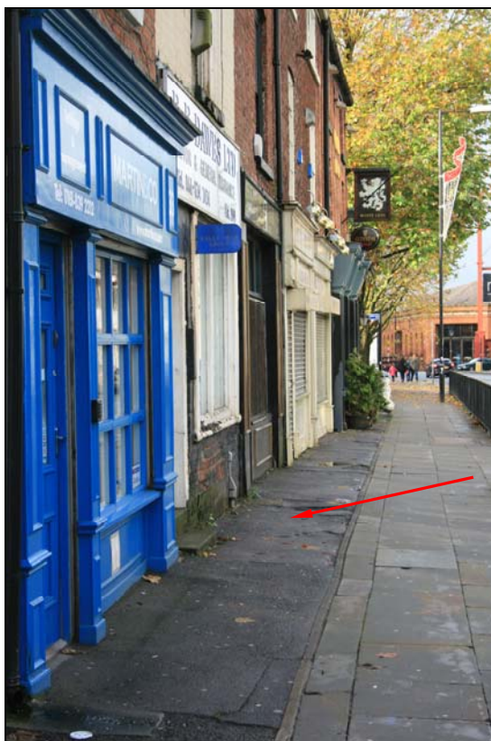
11. Evidence of filled-in basement wells along the front of the row
