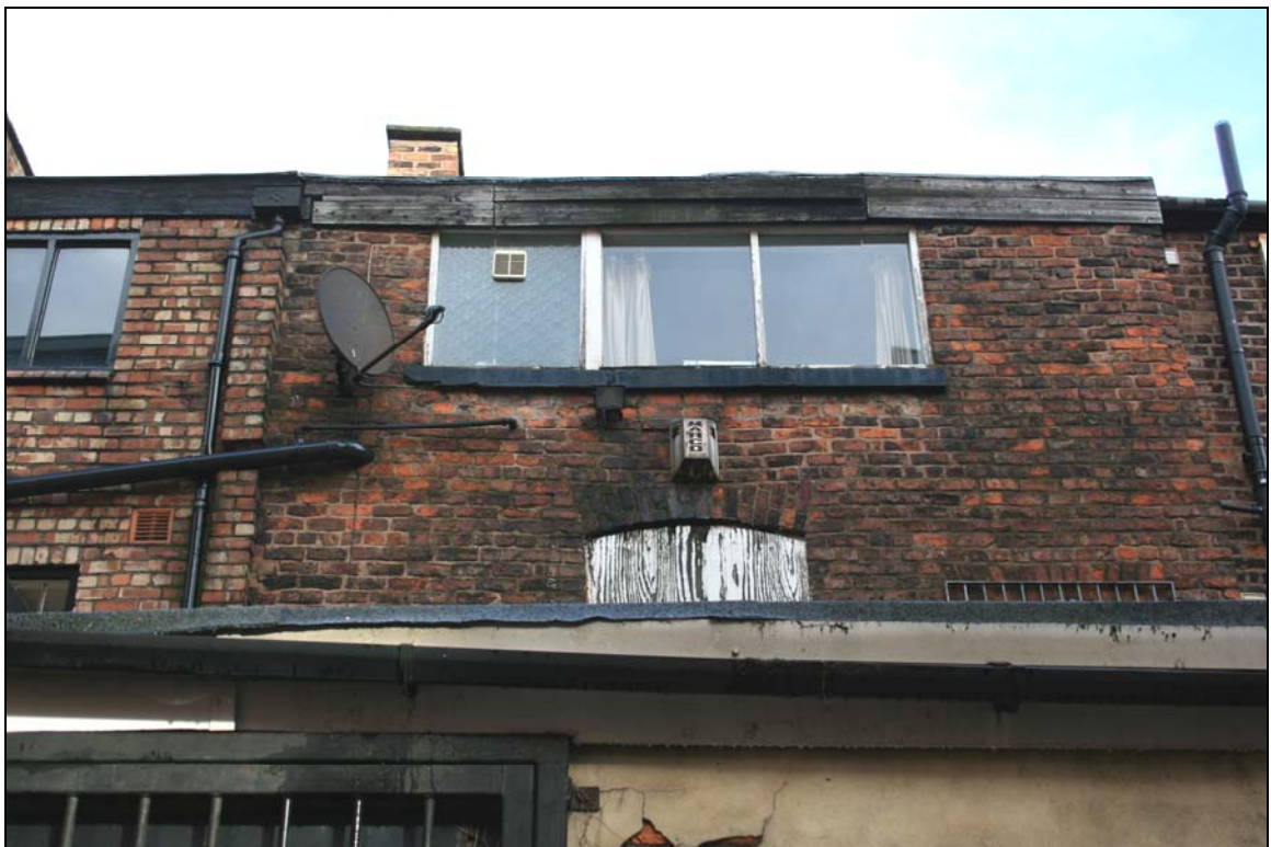
18. Rear, showing first and second floor above single-storey extension
