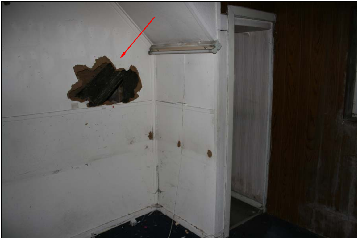
23. Original stair visible through hole in boards at rear of main room
