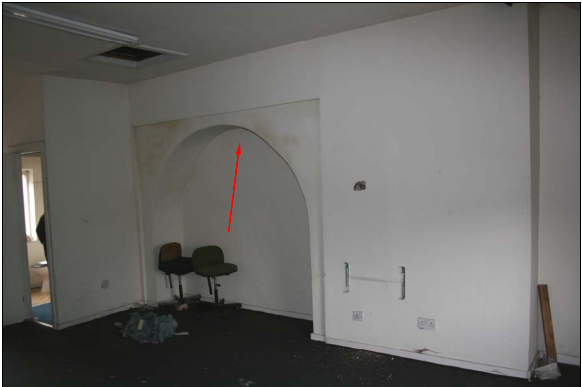
33. Arch formed by converging flues on second floor
