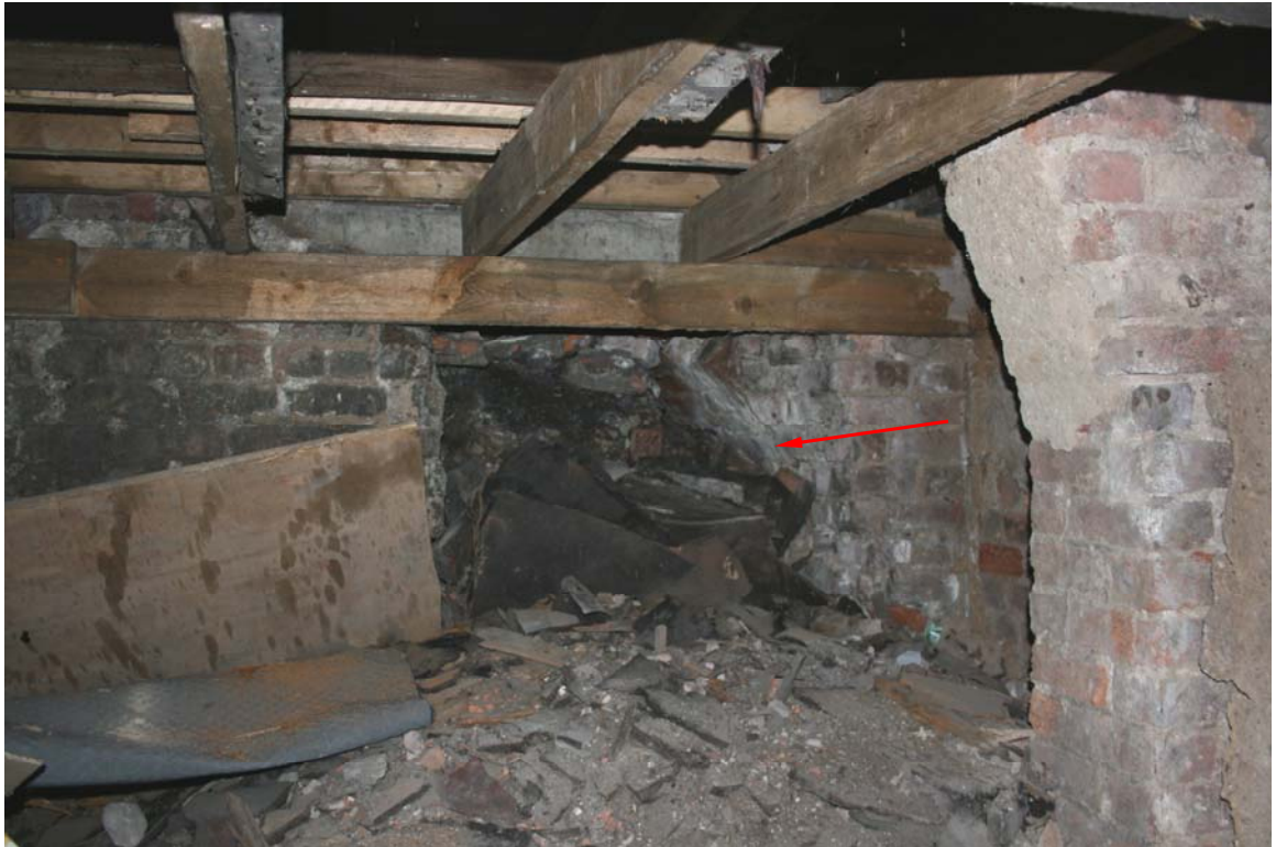
37. Rear room of cellar, looking to space beneath former outrigger (indicated)
