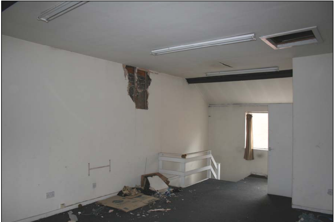
31. Second floor room; gaps in boarded walls shown original brickwork
