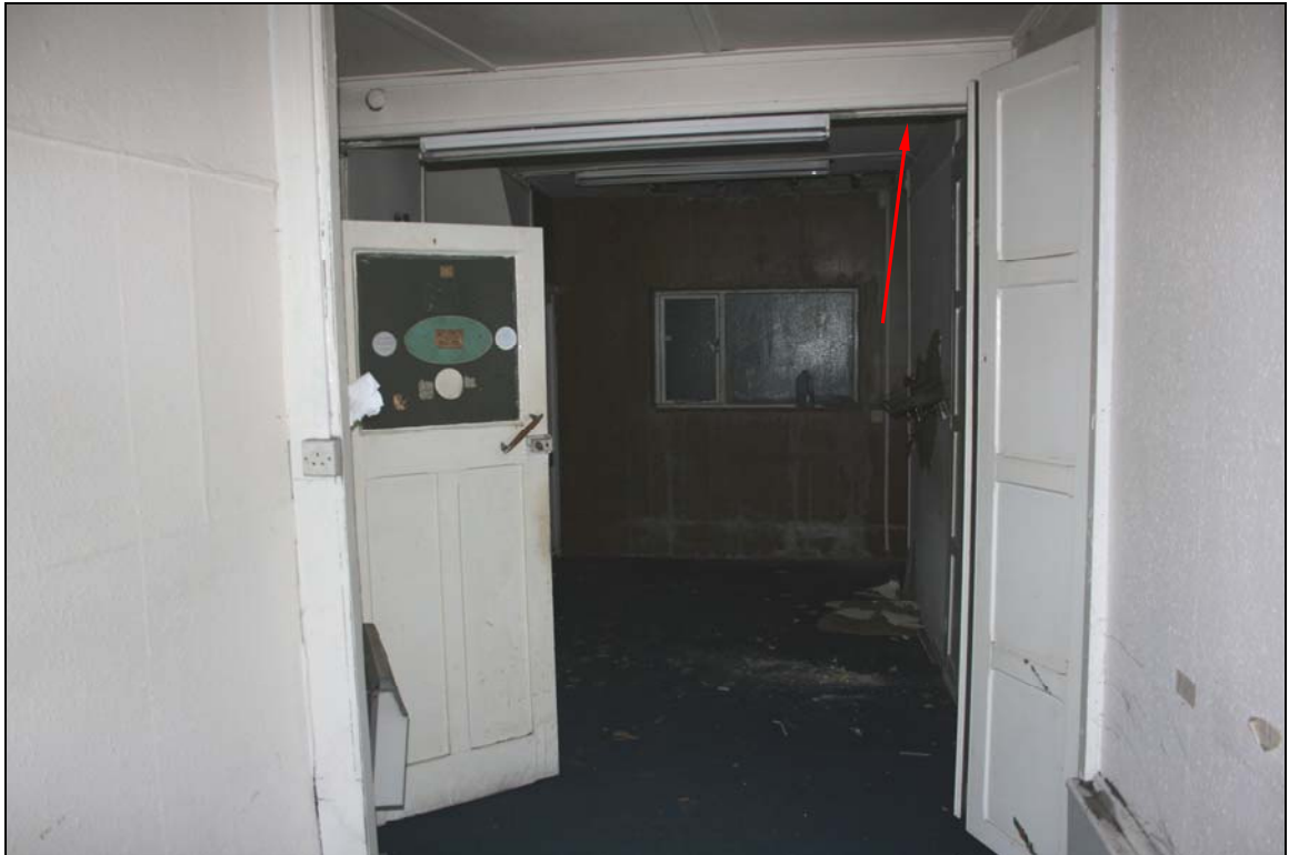
21. Looking to rear of main room showing window to rear extension and line of original crosswall (indicated)
