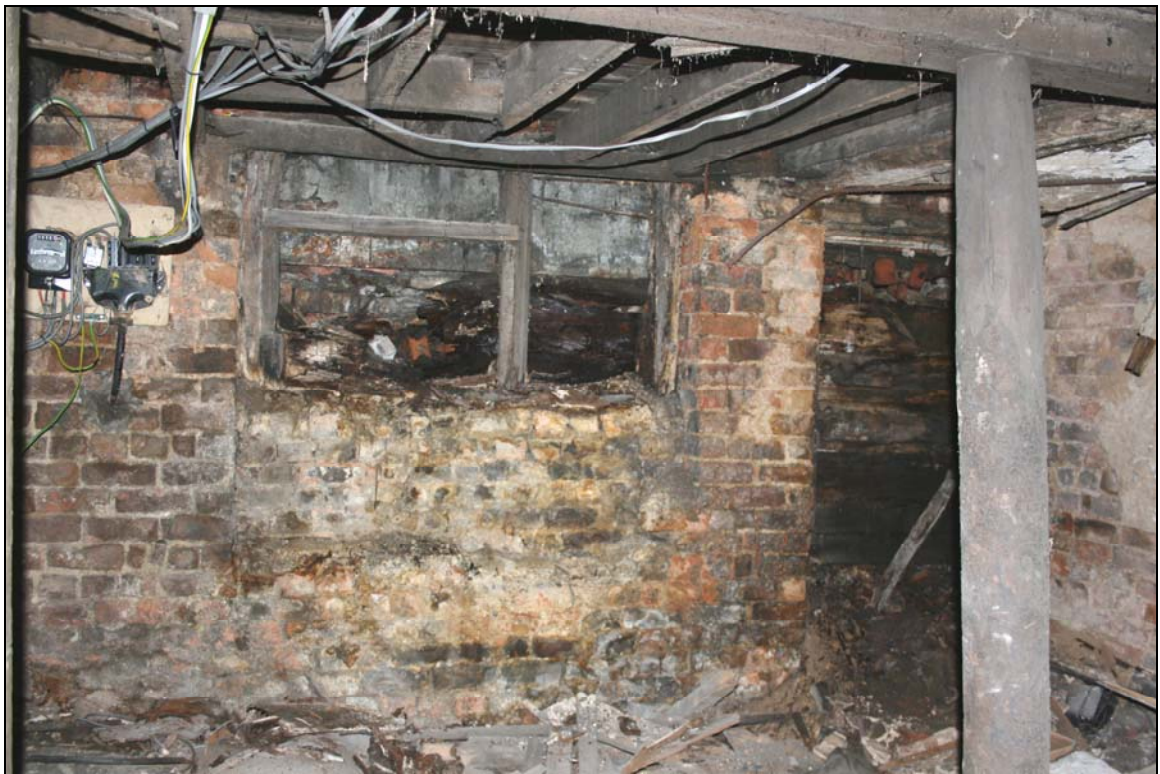
38. Front room of cellar showing window and external door to former steps from street level
