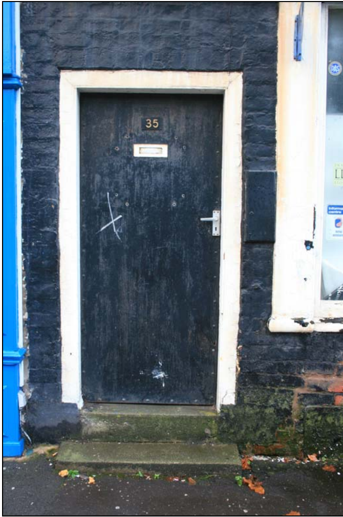
12. Boarded modern doorway in plain architrave
