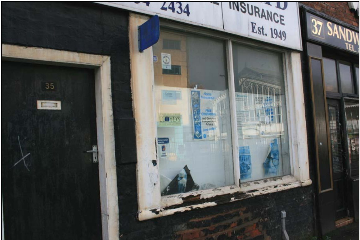
17. The shop window is probably early 20 th century; black paint conceals brickwork
