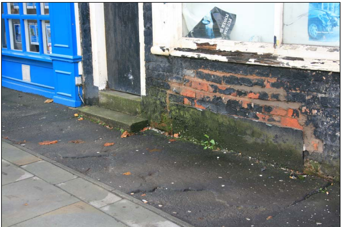
13. Location of basement window and filled-in well in front of the premises
