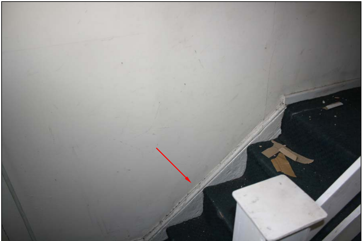
27. Second flight of stair landing to first floor showing original/early skirting; stair is modern
