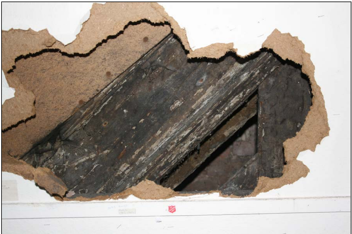
24. Detail of stair
