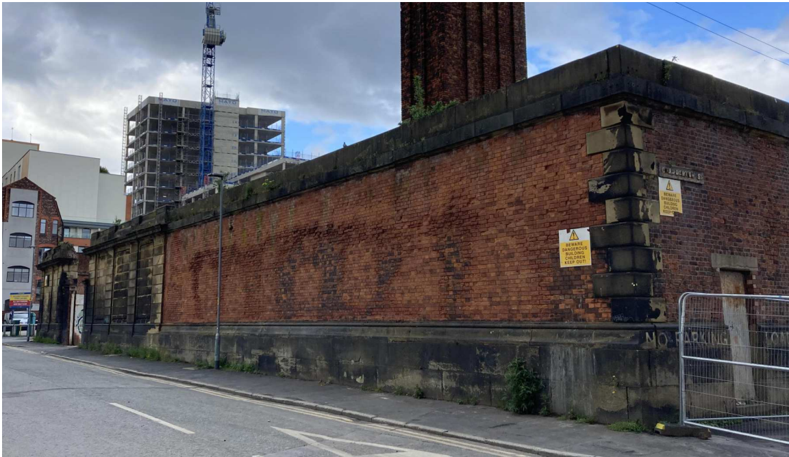
OUTSIDE ELEVATION - EAST END Wall to be partly demolished. East wall corner to be retained and restored.
