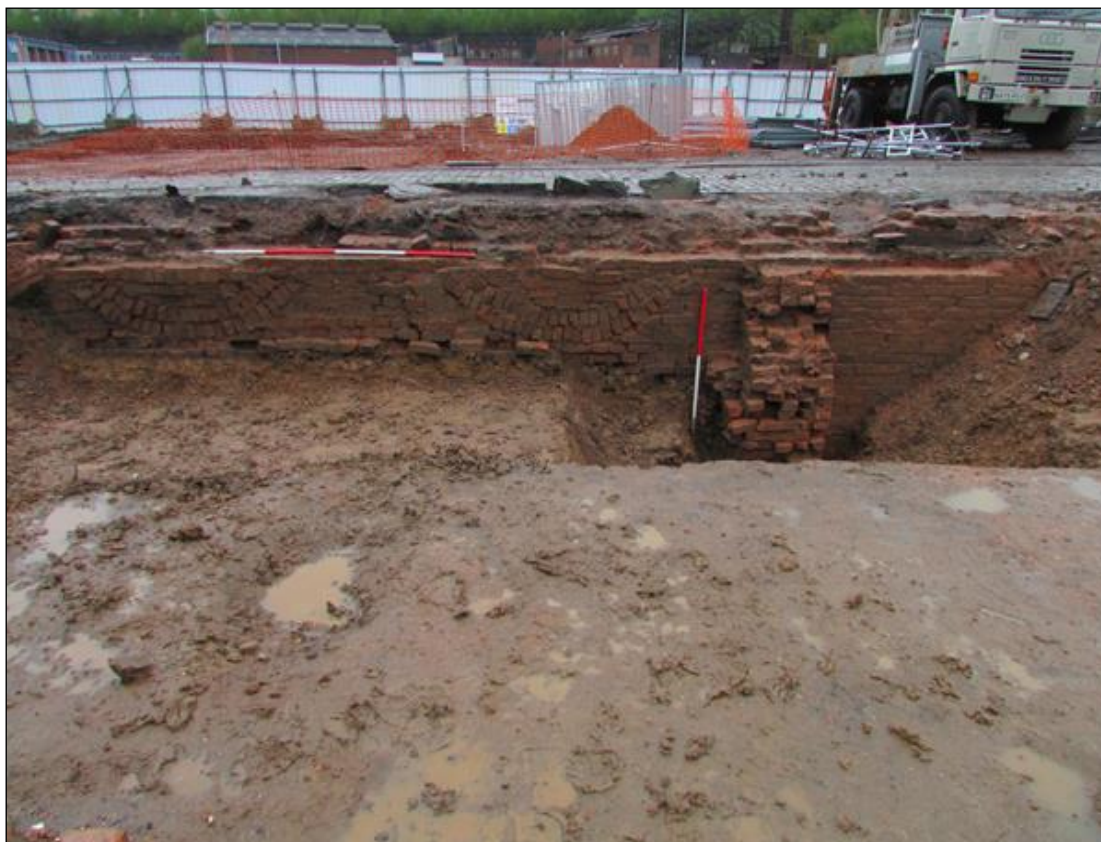
Plate 9: Area B showing Phase One walls 618 and 621 with Phase Two wall 619 to the right, looking north-west.
