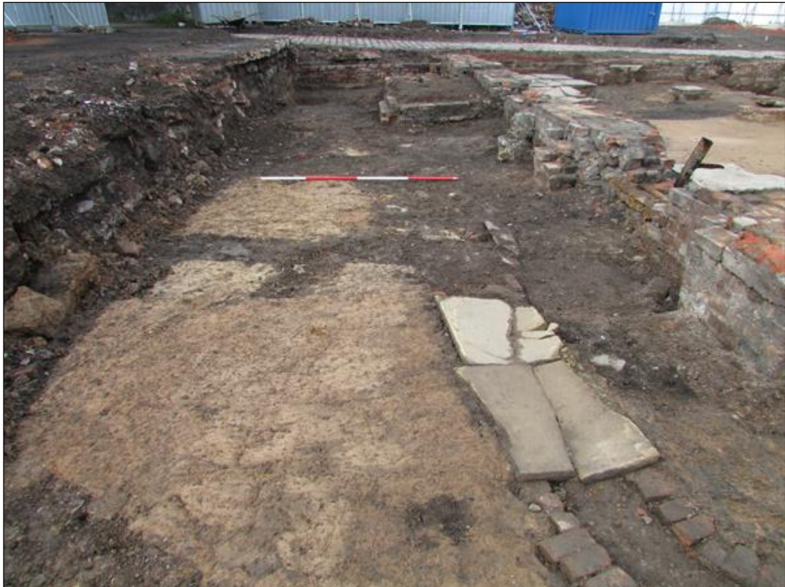
Plate 13: Area B showing drain 609 and area to the east of Parker Street Mill, looking south-west.
