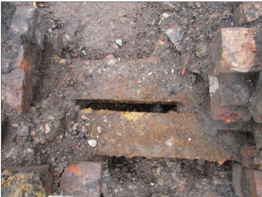
Plate 14: Area B overhead of reinforcing girders 604 within mill wall
