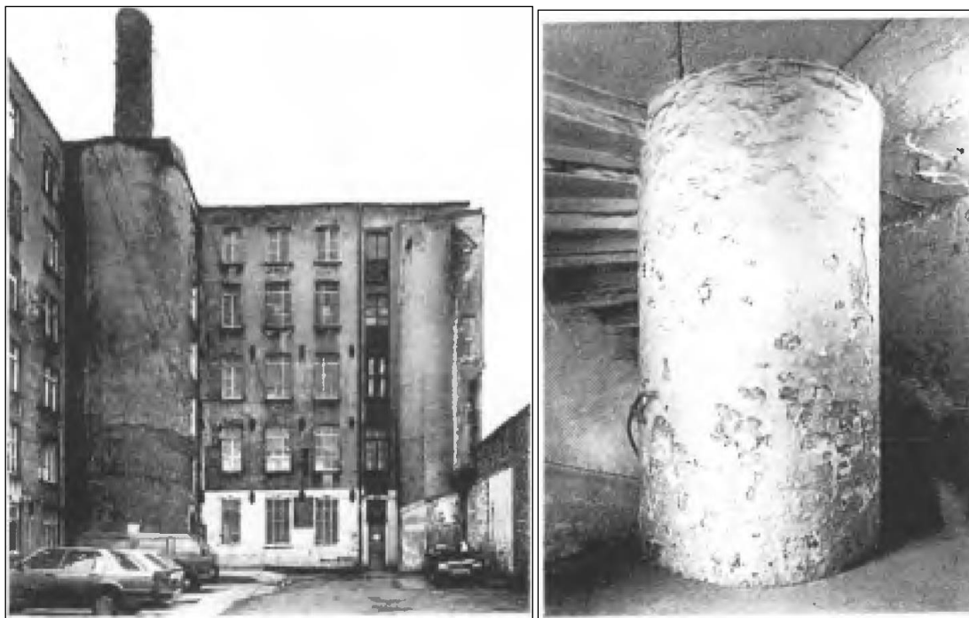
Plate 8: External view (left) and internal view (right) of the extant combined chimney and stair tower at Brownfield Mill, Ancoats, Manchester. Image reproduced with permission from British Brick Society Information 113 July 2010, 4.
