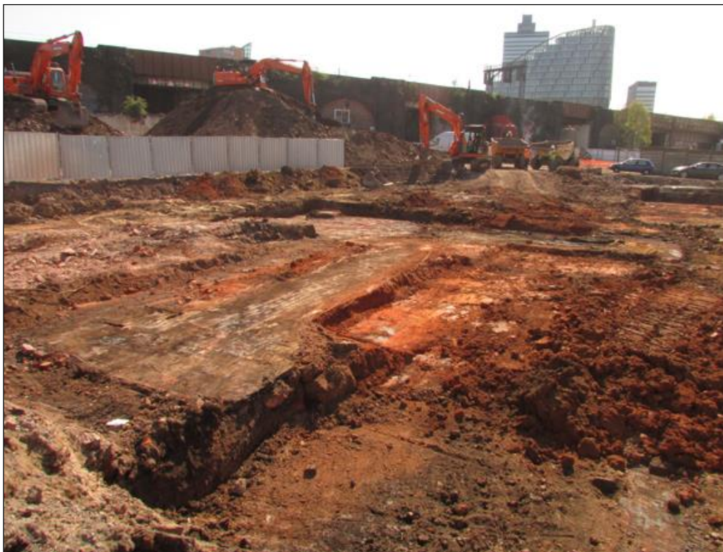
Plate 27: Area A looking south-west.
