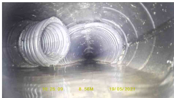
4, 00:00:59, 8.56 m Junction at 9 o'clock, 150mm dia
