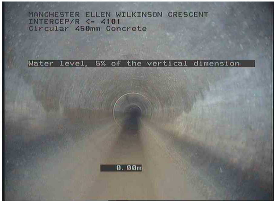
INTERCEP_RX_194de98b-e51d-4379-93d6-334079b5f439_20210528_084439_283.jpg, 00:00:04, 0.00 m Water level, 5% of the vertical dimension
