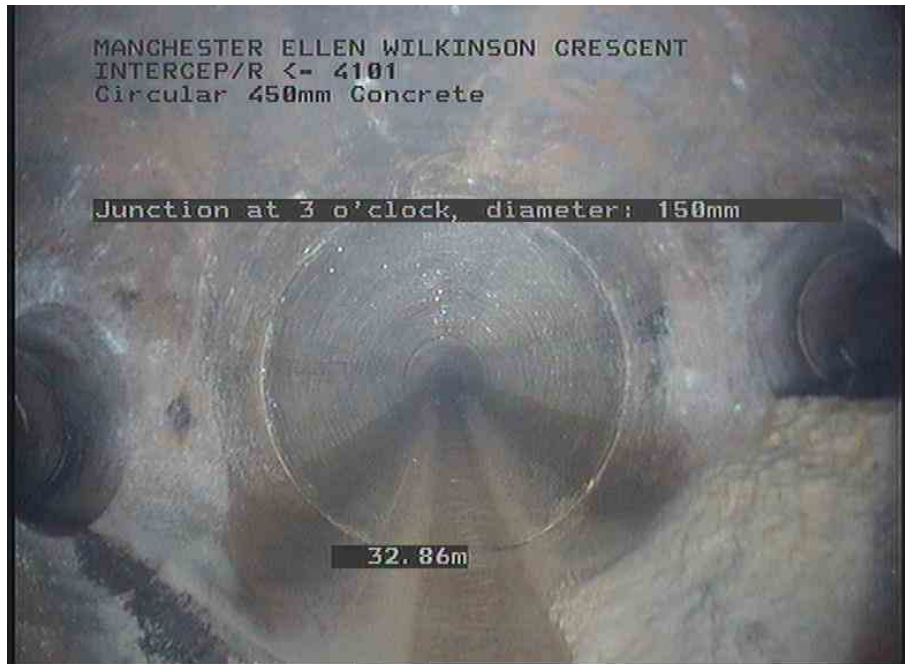
INTERCEP_RX_f6d7f7cb-5dd1-47cf-b30e-0568daee0fad_20210528_084832_815.jpg, 00:03:21, 32.86 m Junction at 3 o'clock, diameter: 150mm
