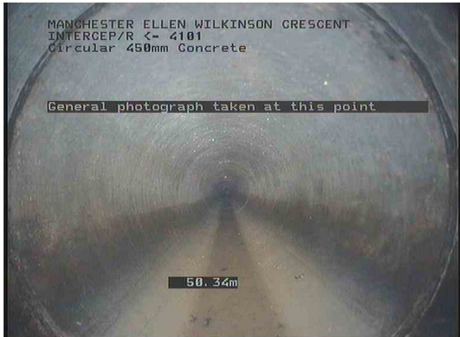
INTERCEP_RX_4def1fbd-323b-409a-aaea-c79f1b9cb3b9_20210528_085019_045.jpg, 00:04:49, 50.34 m General photograph taken at this point
