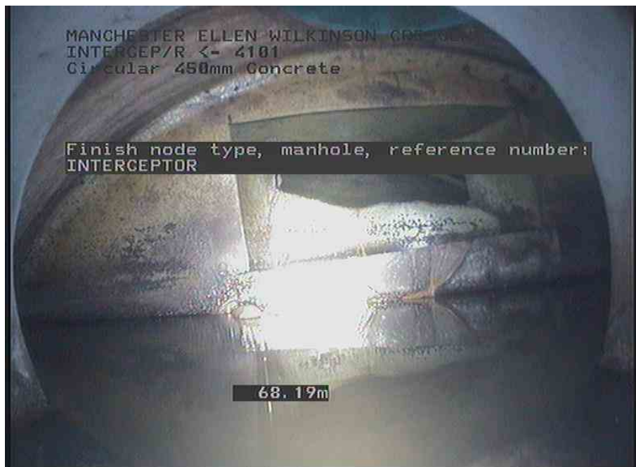
INTERCEP_RX_fc4a4c18-5b76-43fb-8716-3fbc42e12d4b_20210528_085237_815.jpg, 00:06:38, 68.19 m Finish node type, manhole, reference number: INTERCEPTOR
