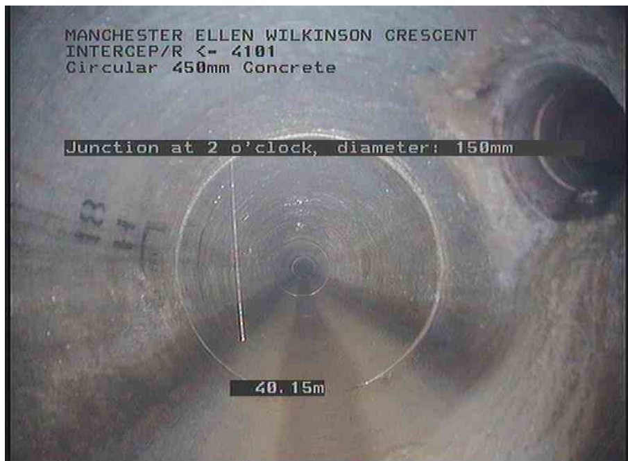
INTERCEP_RX_cd6b0d6c-0e6d-47eb-a074-e3ba2ef13056_20210528_084932_089.jpg, 00:04:05, 40.15 m Junction at 2 o'clock, diameter: 150mm
