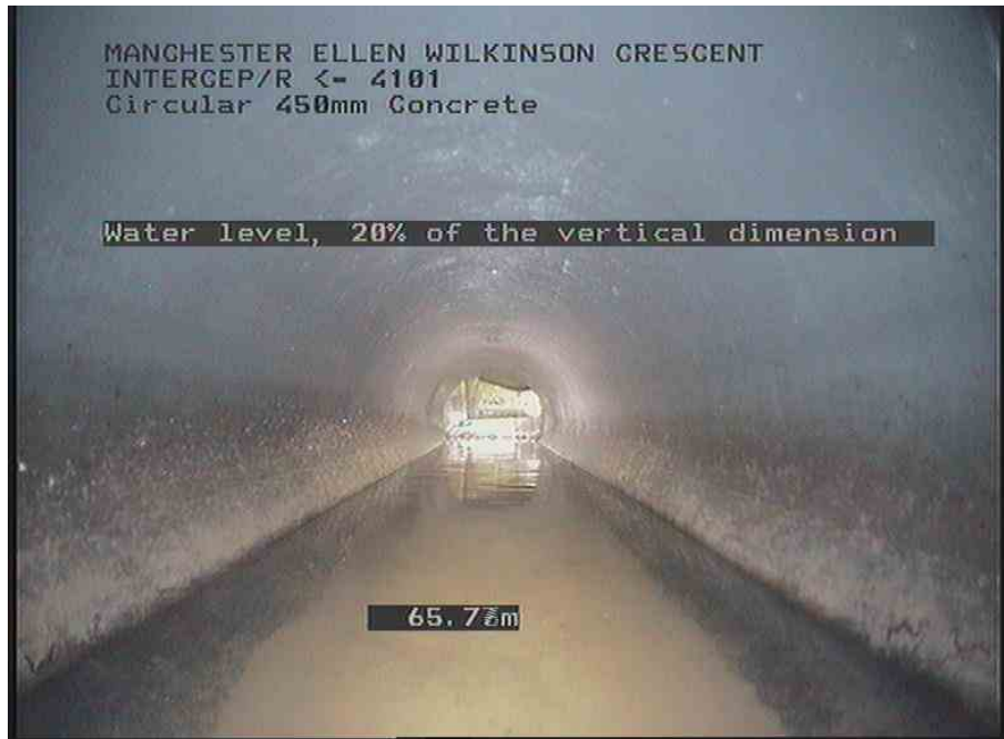
INTERCEP_RX_10a5e499-ca44-4d13-8560-51b7bd231790_20210528_085203_547.jpg, 00:06:17, 66.59 m Water level, 20% of the vertical dimension
