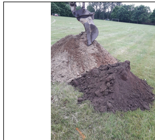
Trial Pit 109 Spoil
