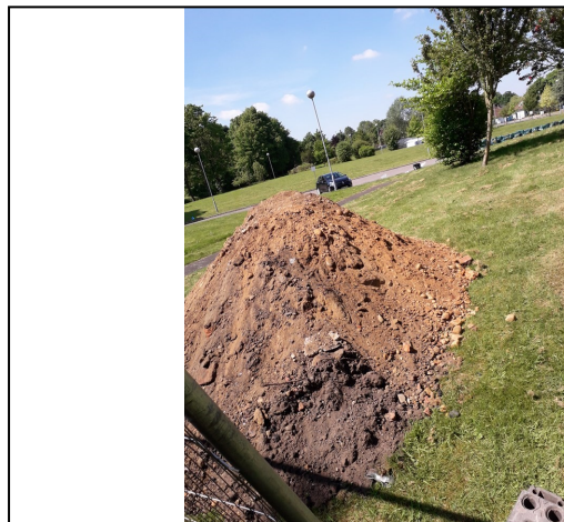
Trial Pit 105/ Soakaway 105 Spoil
