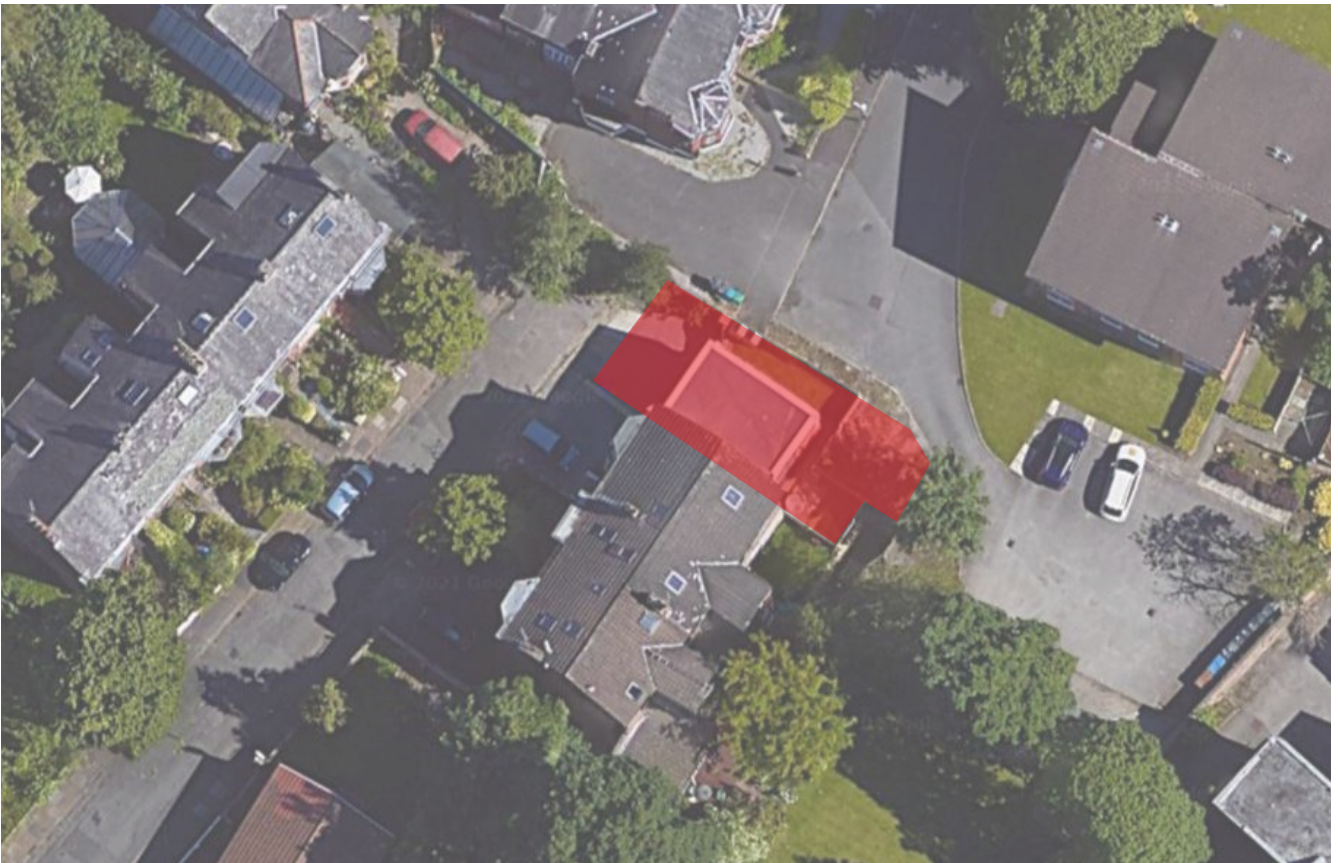
Aerial view of the application site
