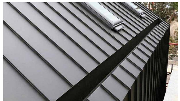
Black standing seam roof and wall cladding
