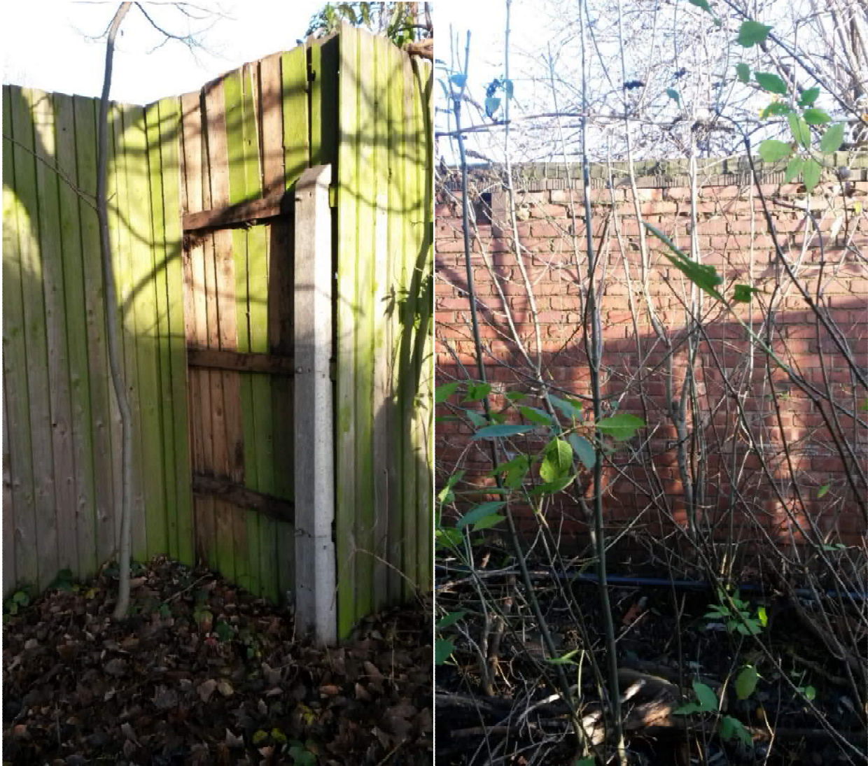
PLATE 1 – BOUNDARY FENCE FACING NORTH WEST, LOOKING NORTHWEST (LHS) PLATE 2 - BOUNDARY WALL FACING NORTH EAST, LOOKING NORTH EAST. JAPANESE KNOTWEED CAN BEE SEEN IN THE FOREGROUND OF THE PHOTO (RHS)
