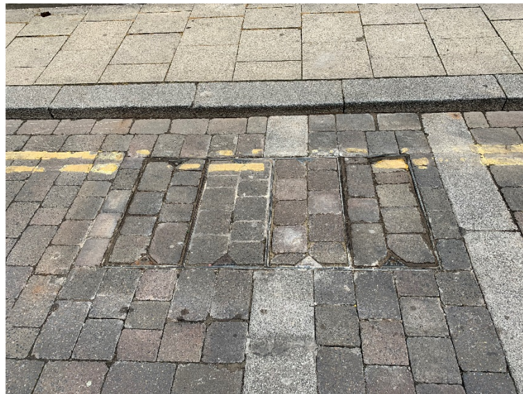
Existing cable chambers in South King Street.
