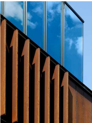
Examples of metal fins with a weathered effect aesthetic
