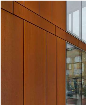
Examples of metal cladding panels with a weathered effect & curtain walling
