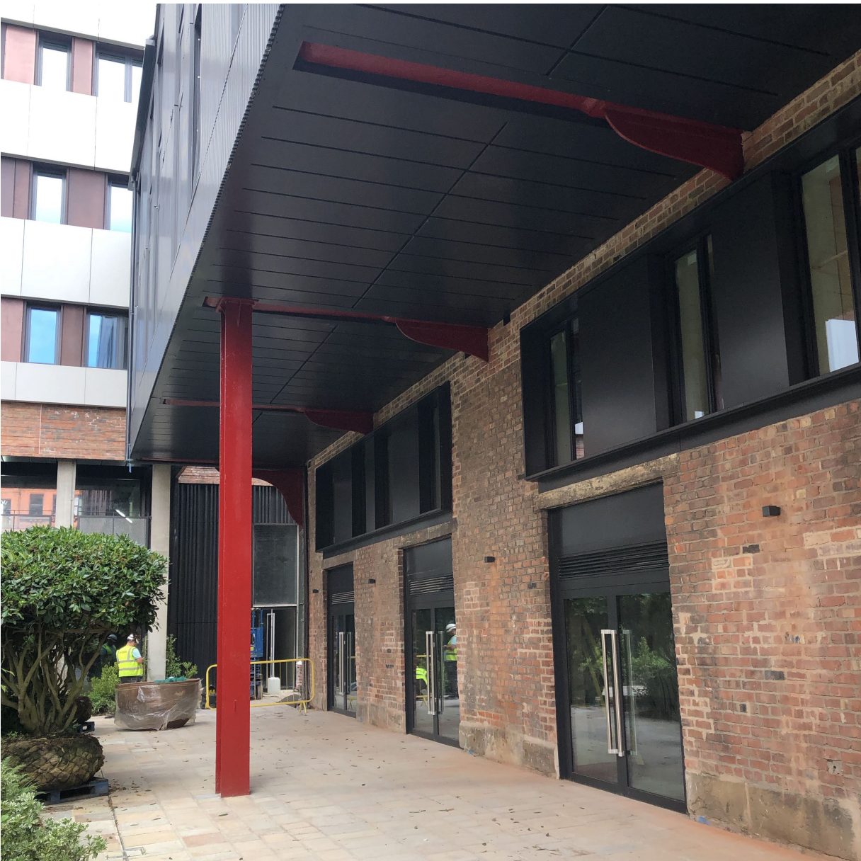
fig 94: minshull house rear elevation (levels 00 + 01) - installation review 14.07.21
