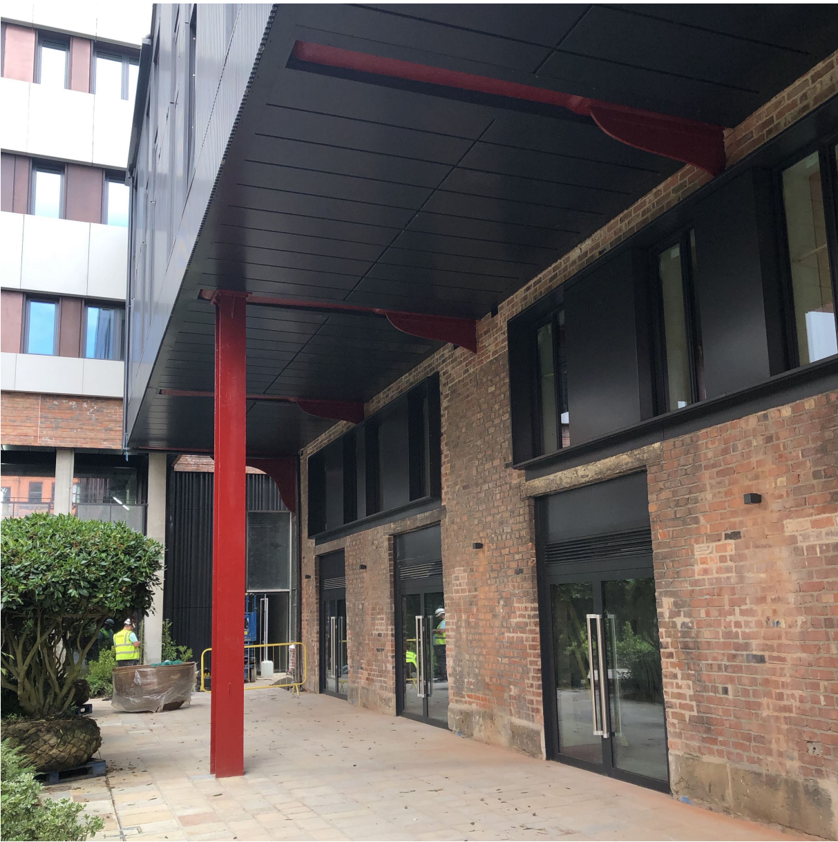
fig 89: minshull house rear elevation (levels 00 + 01) - installation review 14.07.21
