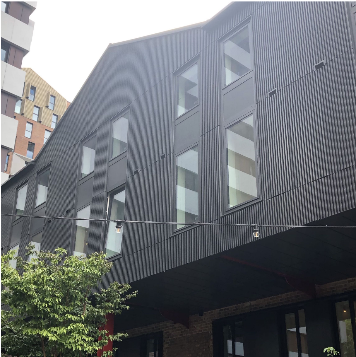
fig 98: minshull house rear elevation (levels 02 + 03) - installation review 14.07.21
