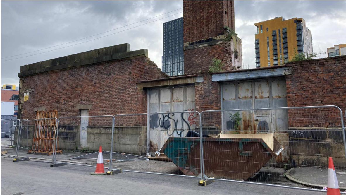
OUTSIDE ELEVATION - MIDDLE PART Sandstone plinth to the left to be retained and restored.
