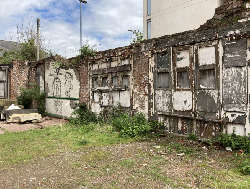
INSIDE ELEVATION - NORTH END Wall to be mainly demolished.
