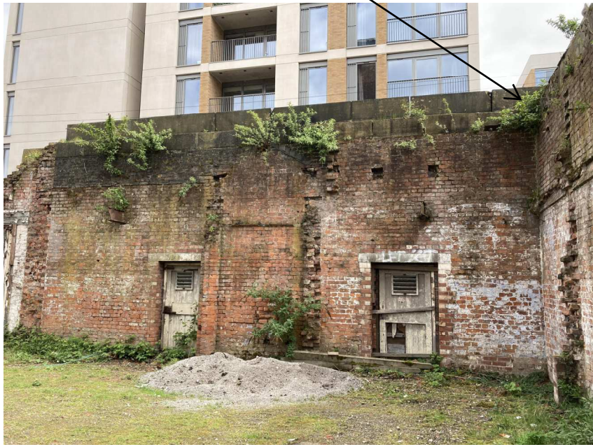
INSIDE ELEVATION - SOUTH END Right corner to be retained and restored.
