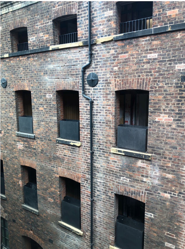
external view of planters + balustrades from minshull house
