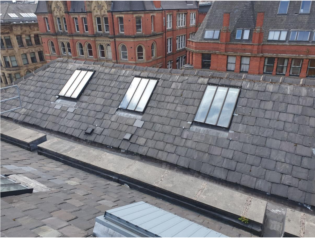
9. Inner slope of hipped roof, note uneven slate courses.
