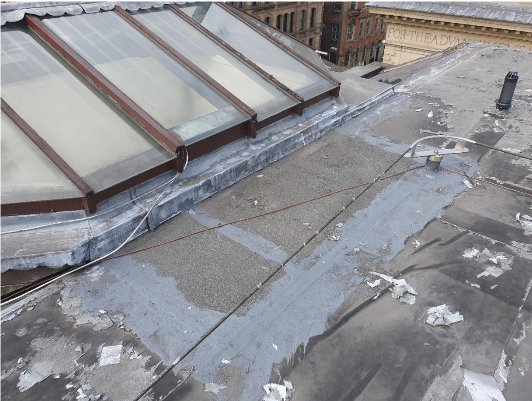
10. Patch repair adjacent to stair atrium.
