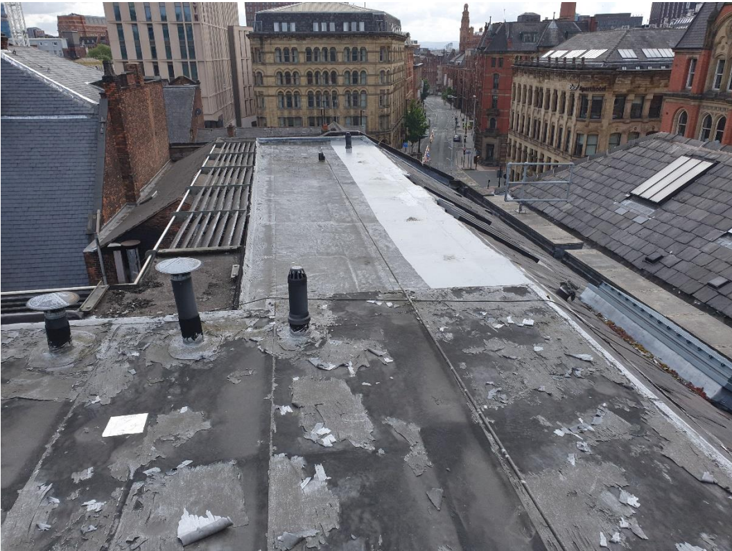
6. Flat roof extending out to side of lightwell.
