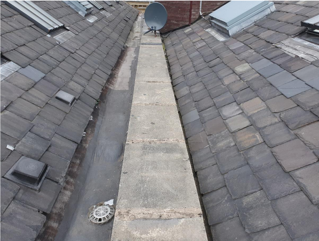
19. Asphalt lined valley between the front pitched roof and mono-pitch roof to the rear section.
