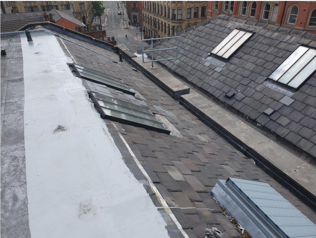
8. Liquid applied patch repair at junction of slate and flat roof.
