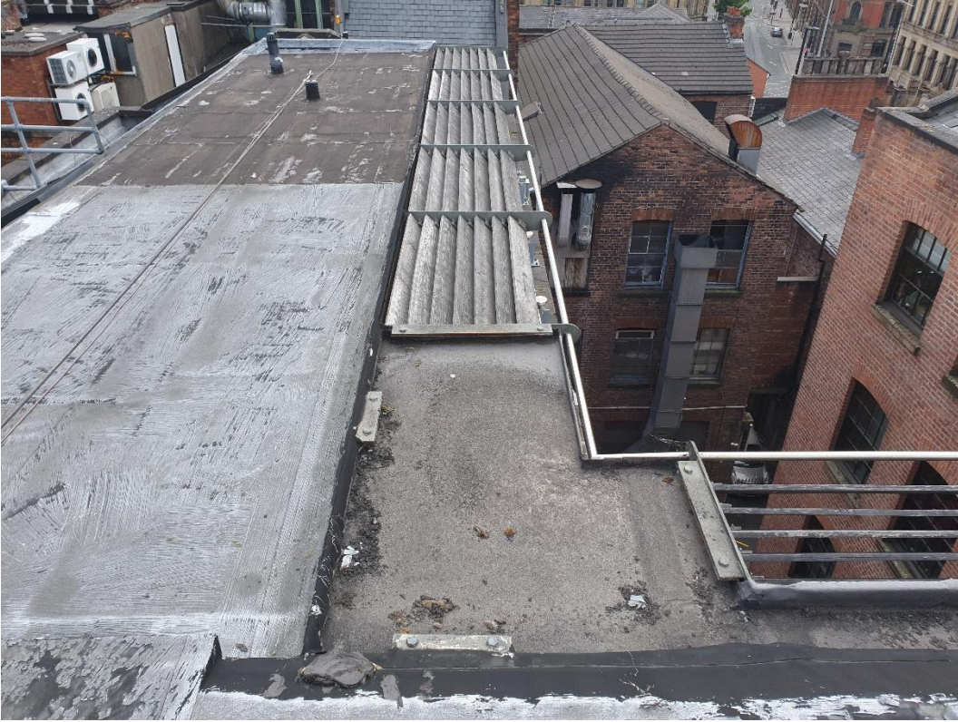
7. Flat roofs and brise-soleil around lightwell
