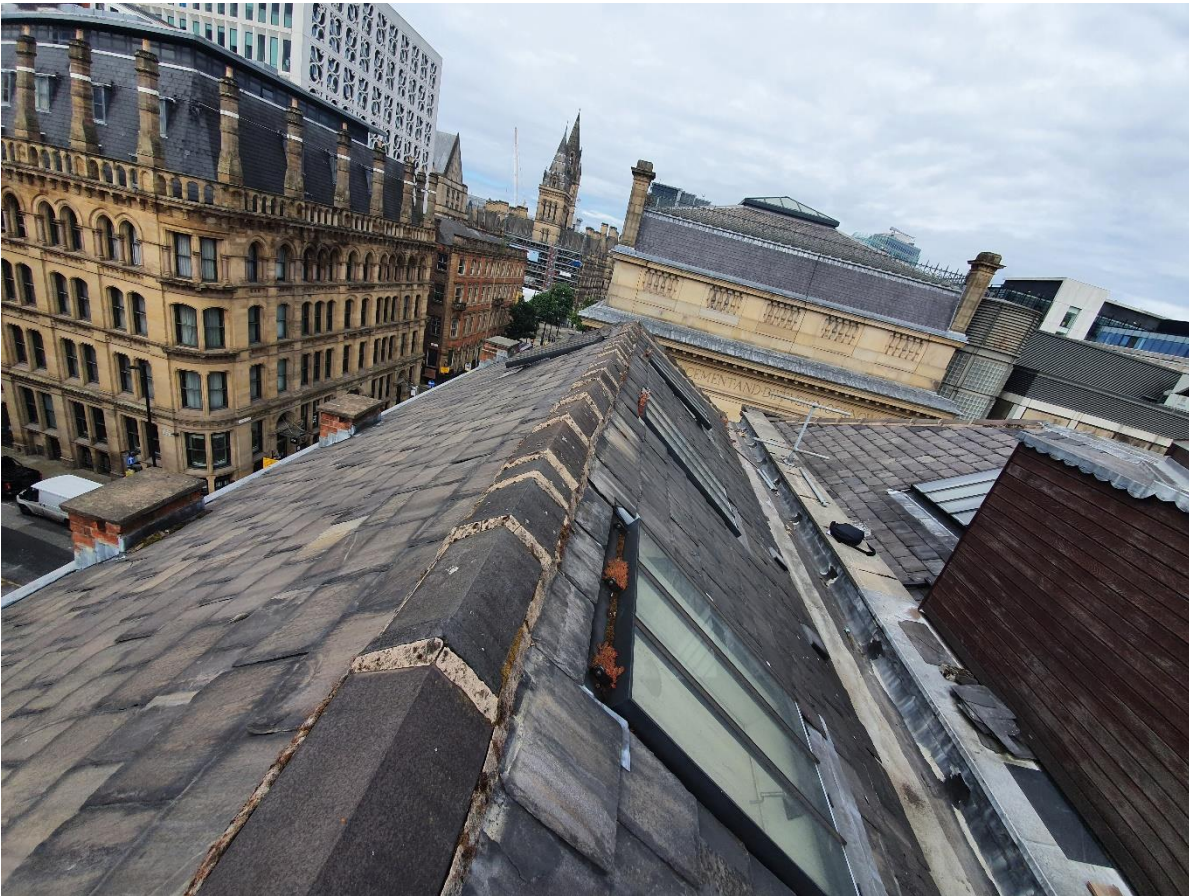
18. Slate covered hipped roof to front section and view of valley.
