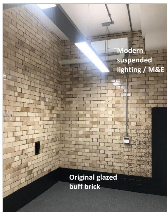
Figure 8 (left): Example of original glazed brick within one of the recessed alcoves to the north wall of the unit. Figure 9 (right): example of original sash windows with deep sill.
