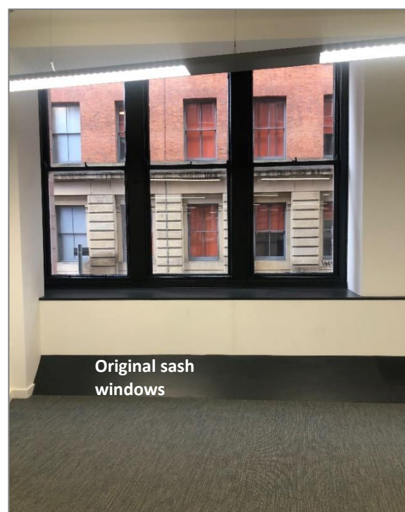
Figure 8 (left): Example of original glazed brick within one of the recessed alcoves to the north wall of the unit. Figure 9 (right): example of original sash windows with deep sill.
