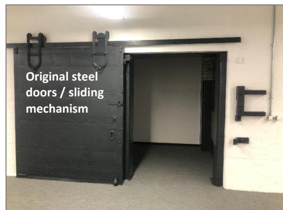
Figure 6 (left): Looking north west across the GF.UI space, illustrating the refurbishment undertaken in 2019 which retains the historic column arrangement and original steel doors. Figure 7 (right): An example of one of the original steel sliding doors.
